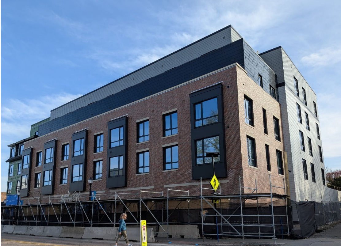
104 Main Street Under Construction
