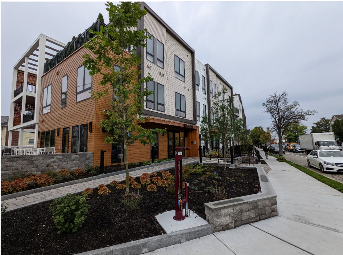
101 North Beacon Street
