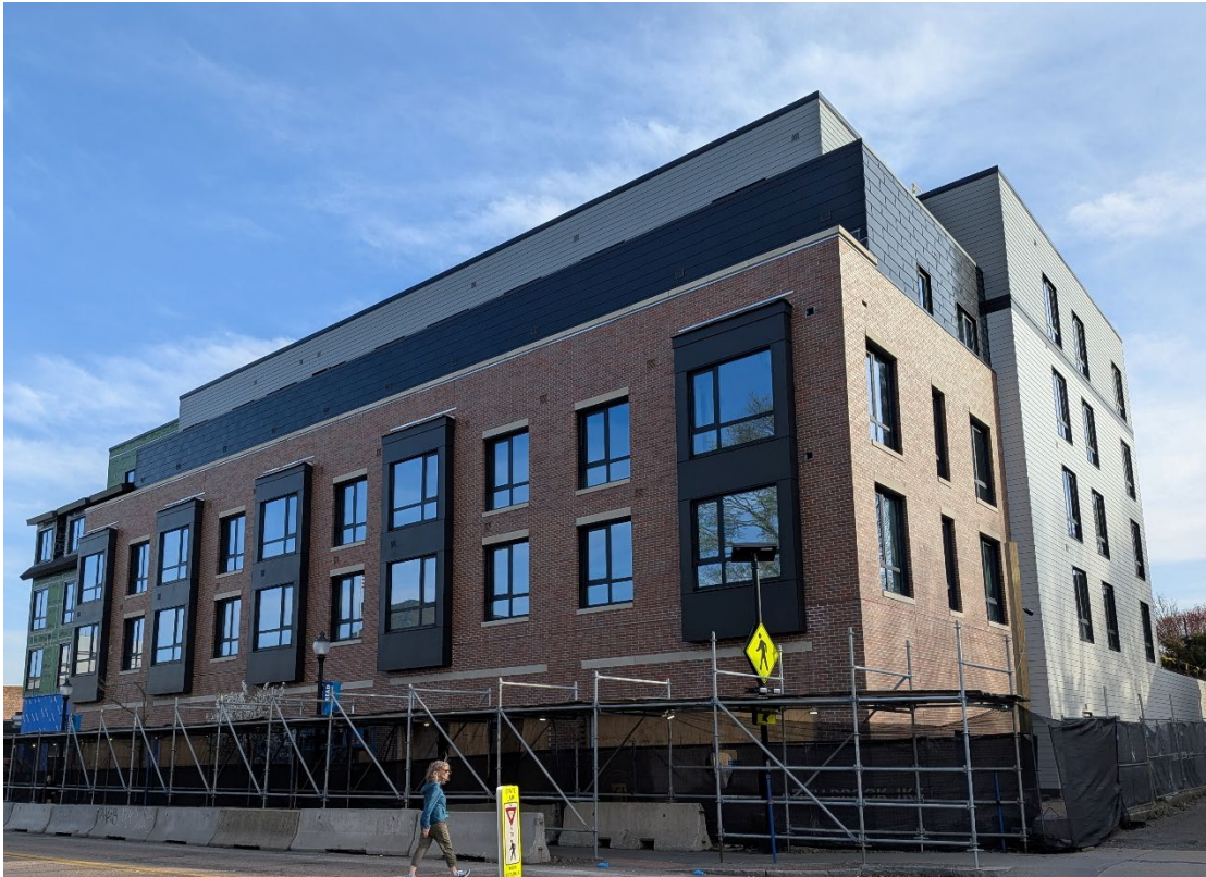
104 Main Street Under Construction
