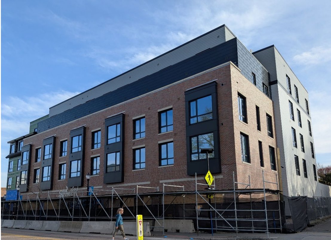
104 Main Street Under Construction
