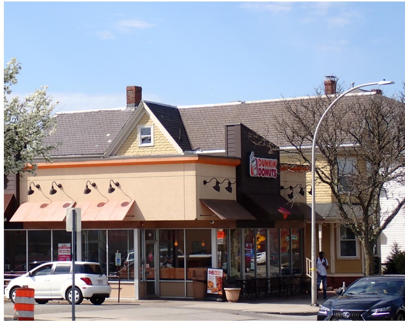
View of roof and east elevation (background). Note mismatched slate repair.
