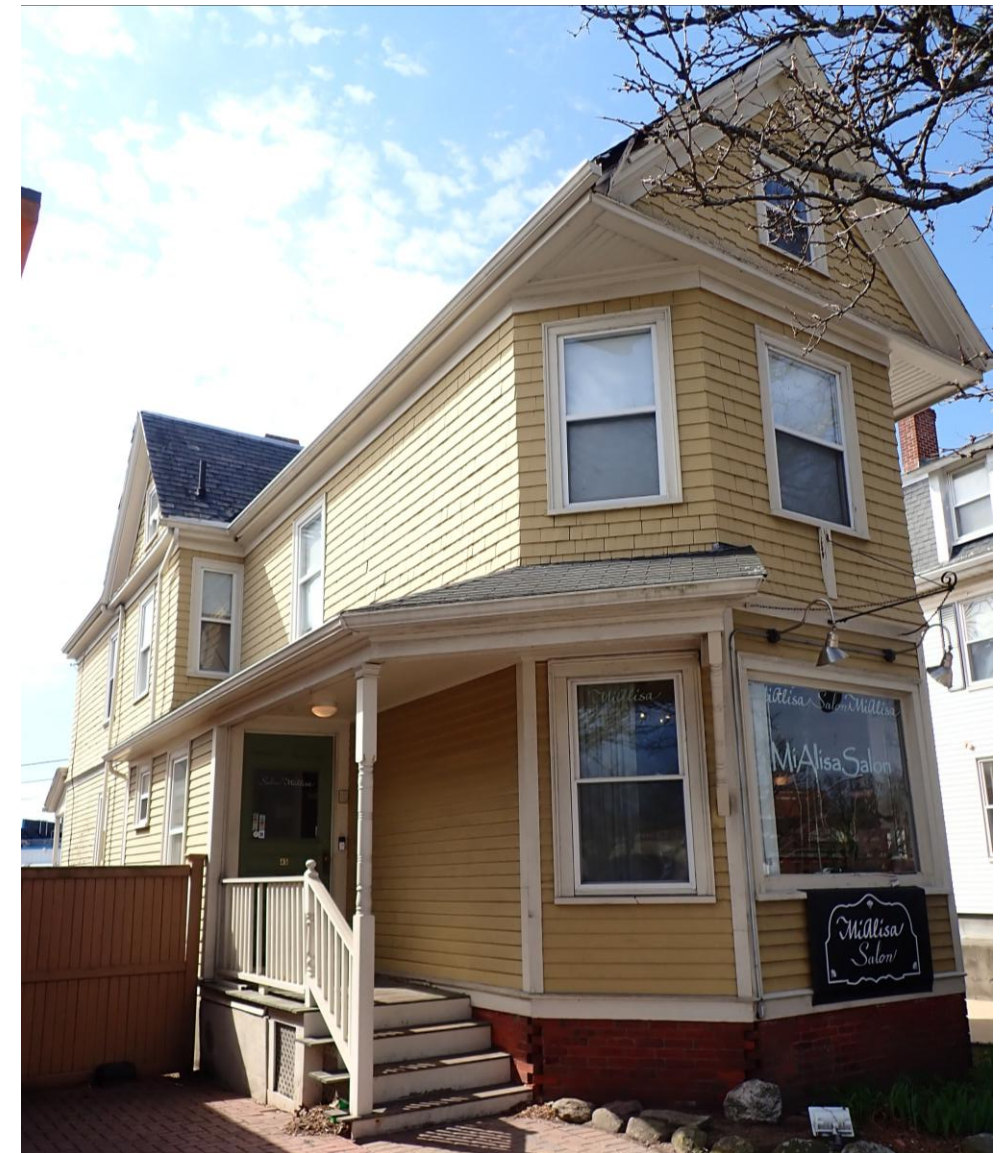
View of façade and east elevation. Note damage at cornice
