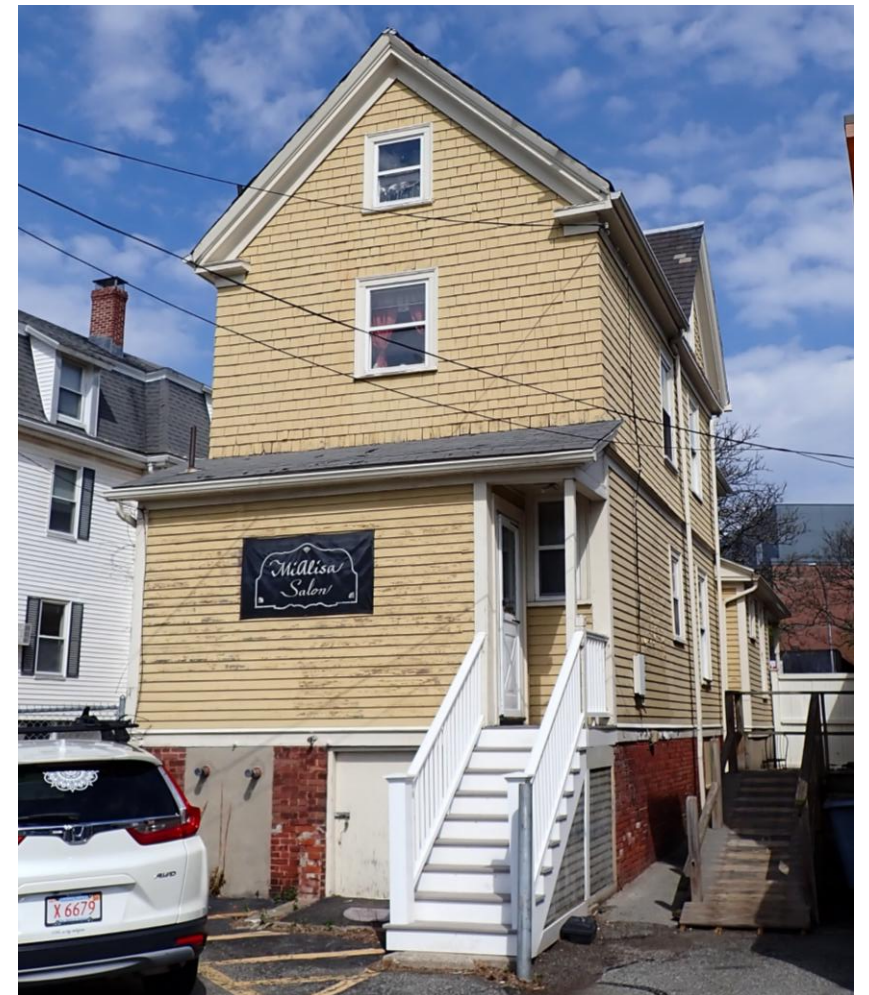
View of rear (south) elevation. Note infill of historic rear porch at first story.
