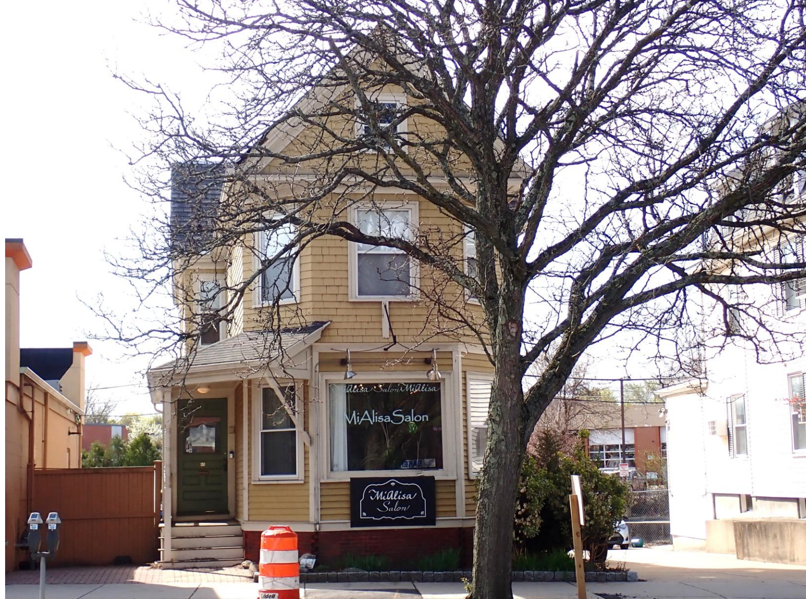
View of façade (north elevation). Note modern display window and replacement windows.
