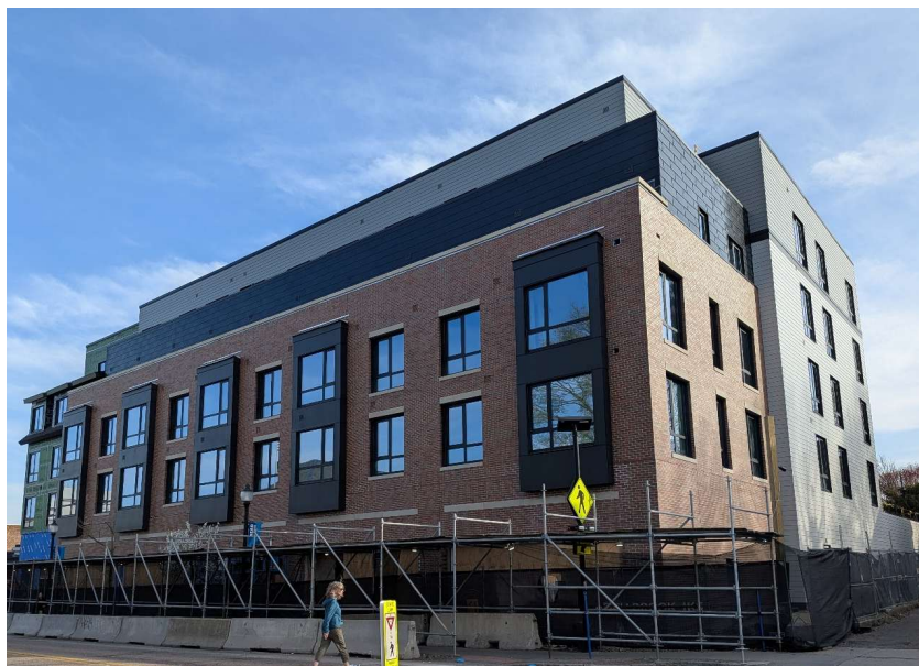
104 Main Street Under Construction
