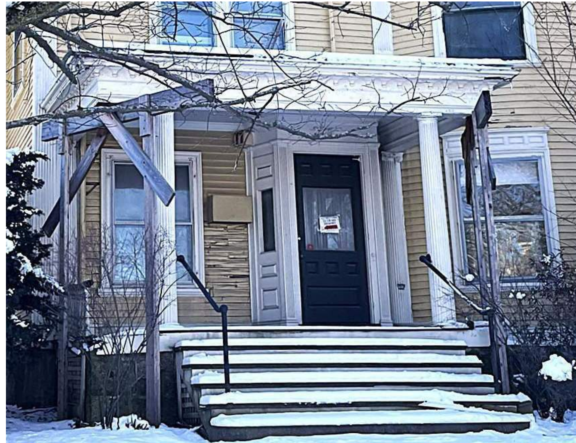
FRONT PORCH DETAIL - MT. AUBURN ST FACADE
