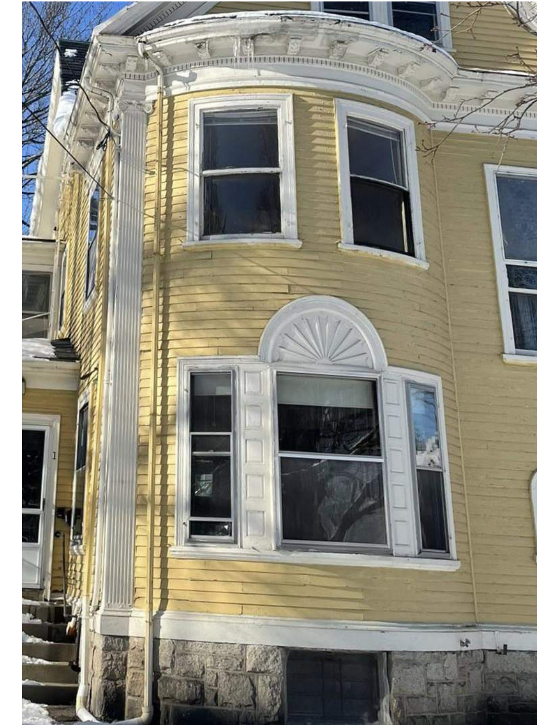
PALLADIAN WINDOW - WALNUT ST FACADE
