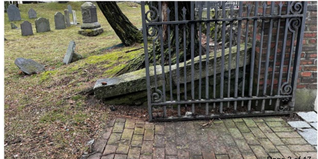
Page 3 of 17 Existing Conditions at Entry Gate
