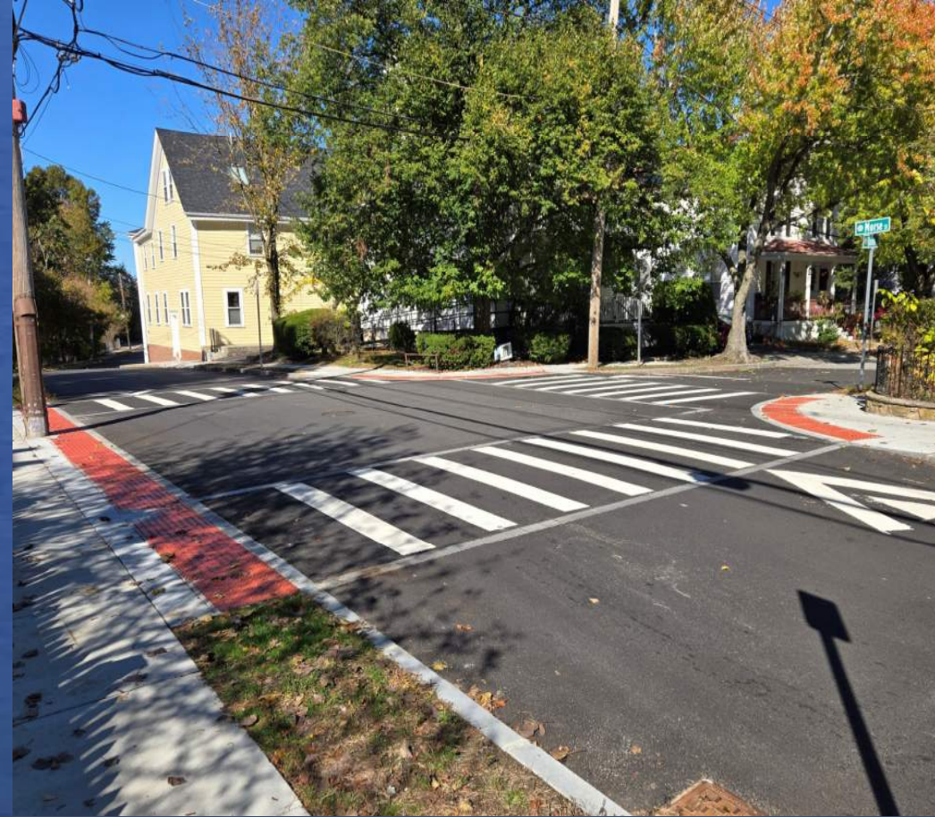
Morse Street - After
