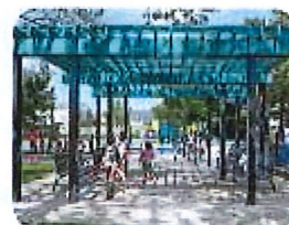
Open Roof Shade Structure
