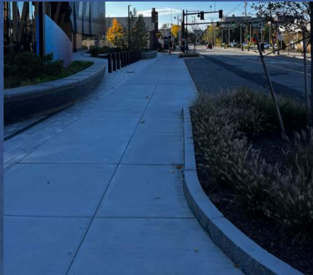
Arsenal St Phase D - After
