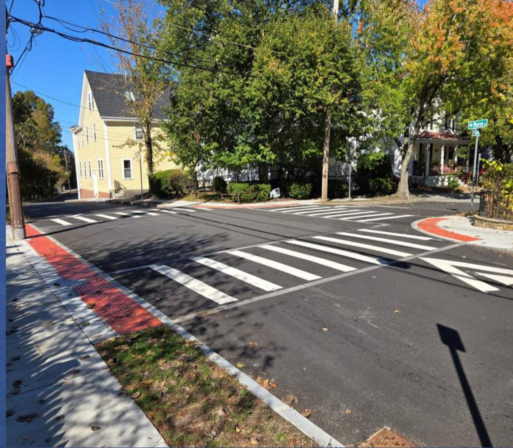
Morse Street - After
