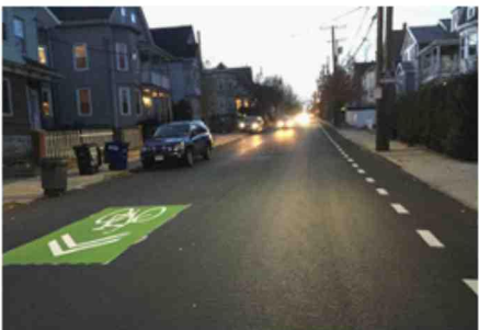
➤ “Super Sharrow” and Advisory Lane – Summer Street, Somerville. These interventions create a comfortable bike environment on lower-volume residential roads in particular
