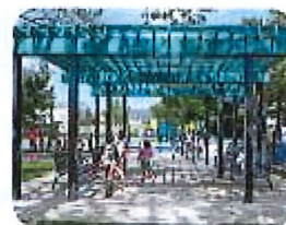
Open Roof Shade Structure
