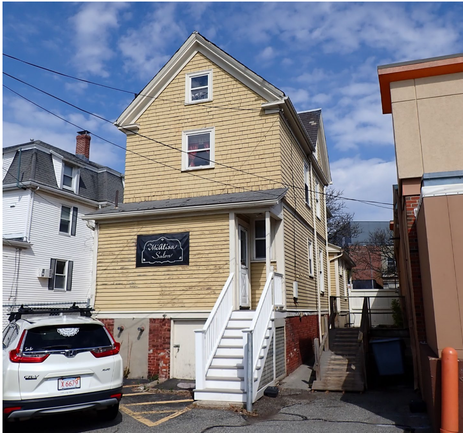
5. View of rear (south) elevation. Note infill of historic rear porch at first story. 41-43 Mt. Auburn Street (left) and 49 Mt. Auburn Street (right).
