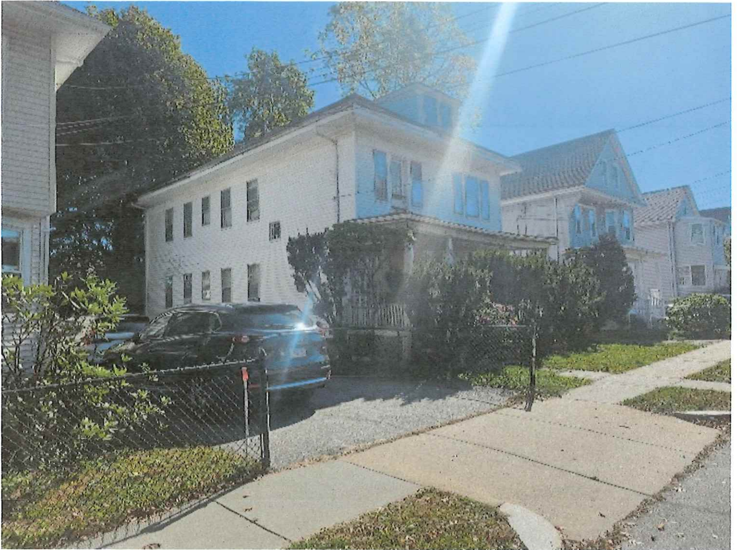
157-159 School Street Northerly
