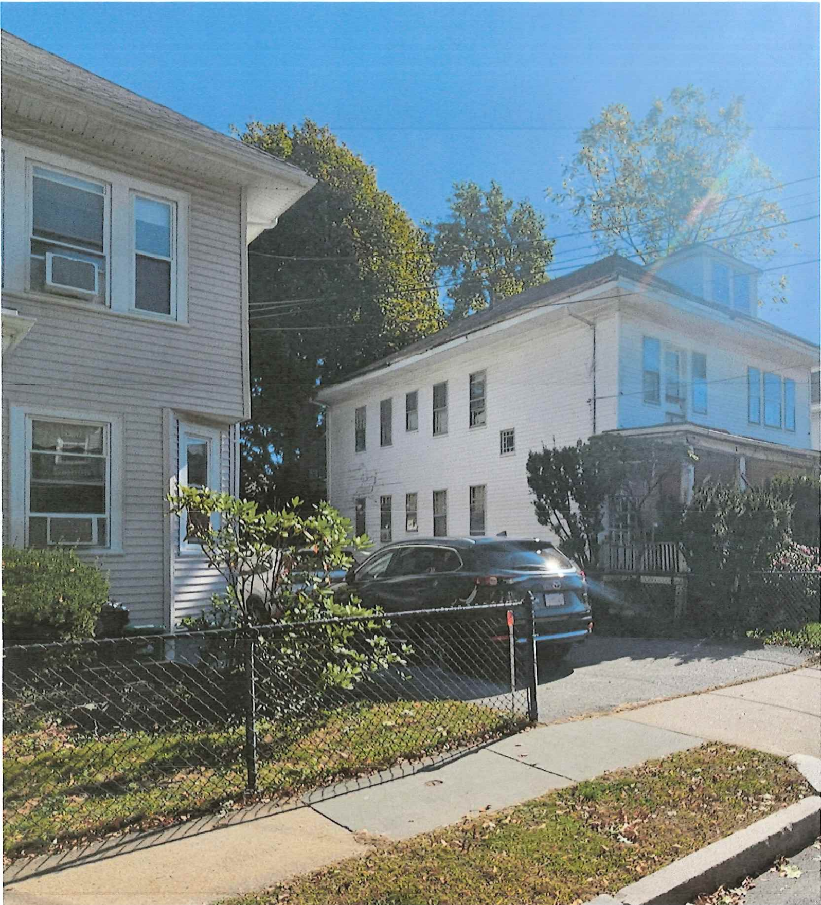
157-159 School Street 161-163 School Street Northerly
