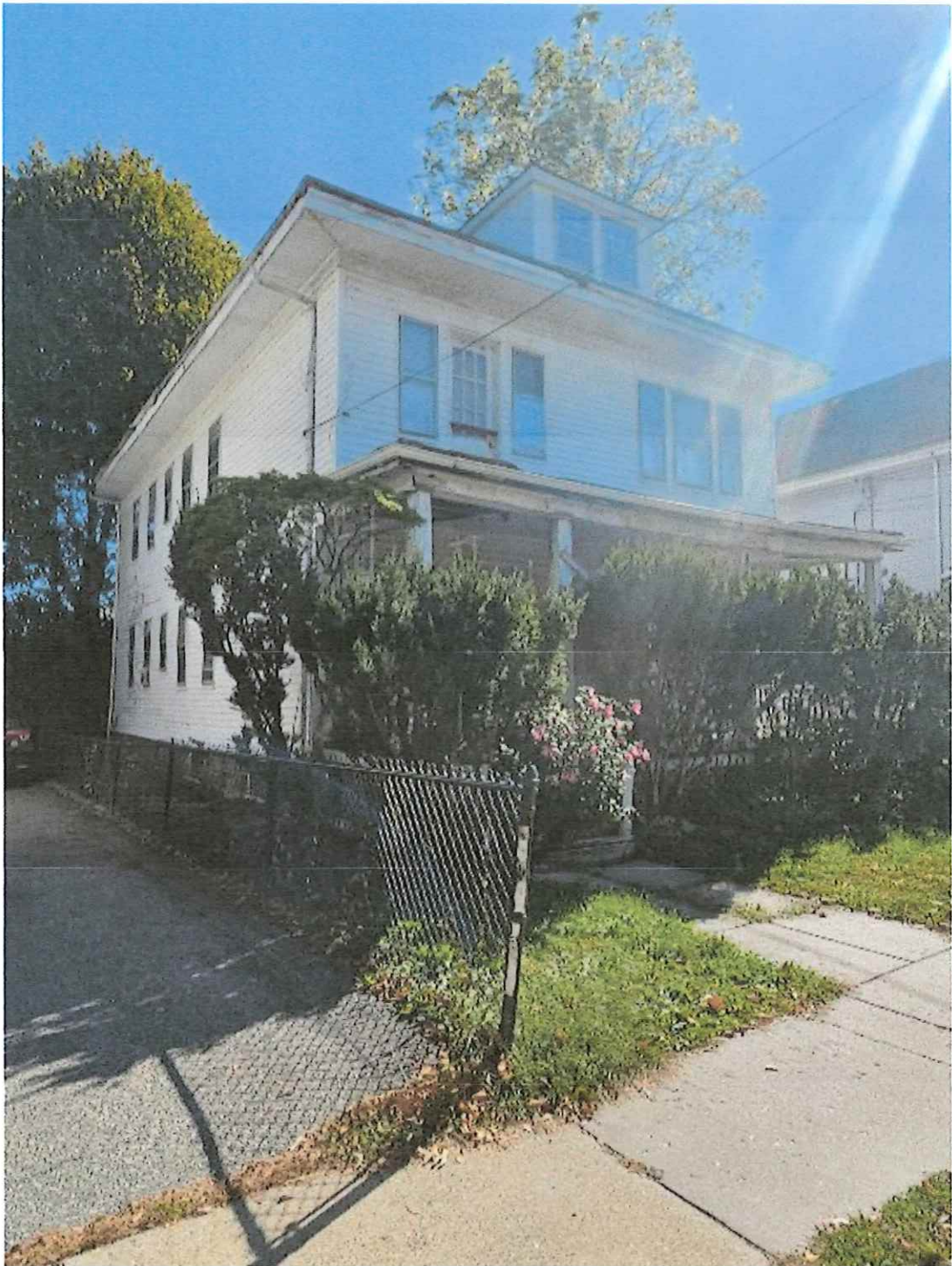
157-159 School Street Northerly
