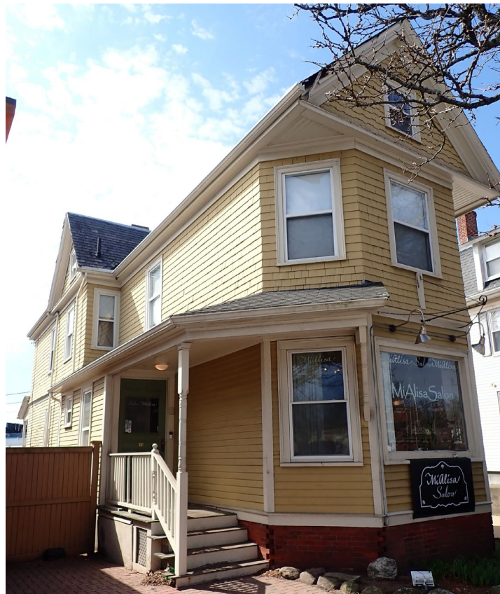
2. View of façade and east elevation of 45 Mt. Auburn Street. Note damage at cornice.
