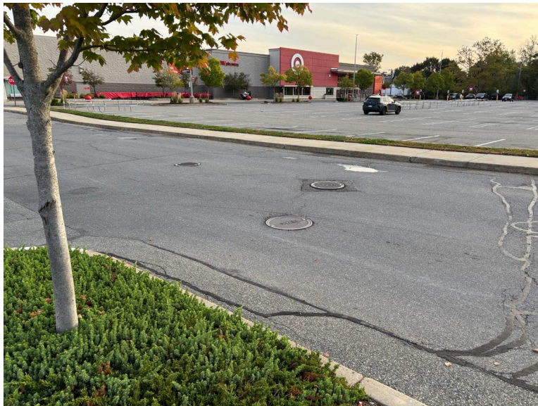
PHOTO #2: Stormwater Improvements In Main Access Driveway
