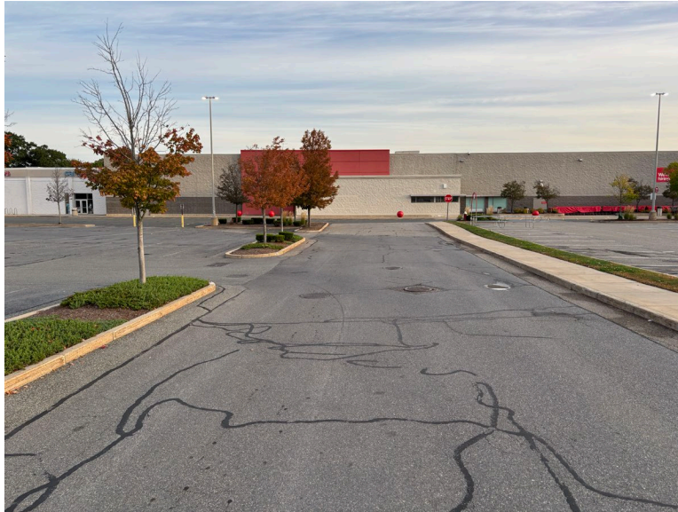
PHOTO #1: Main Access Driveway
