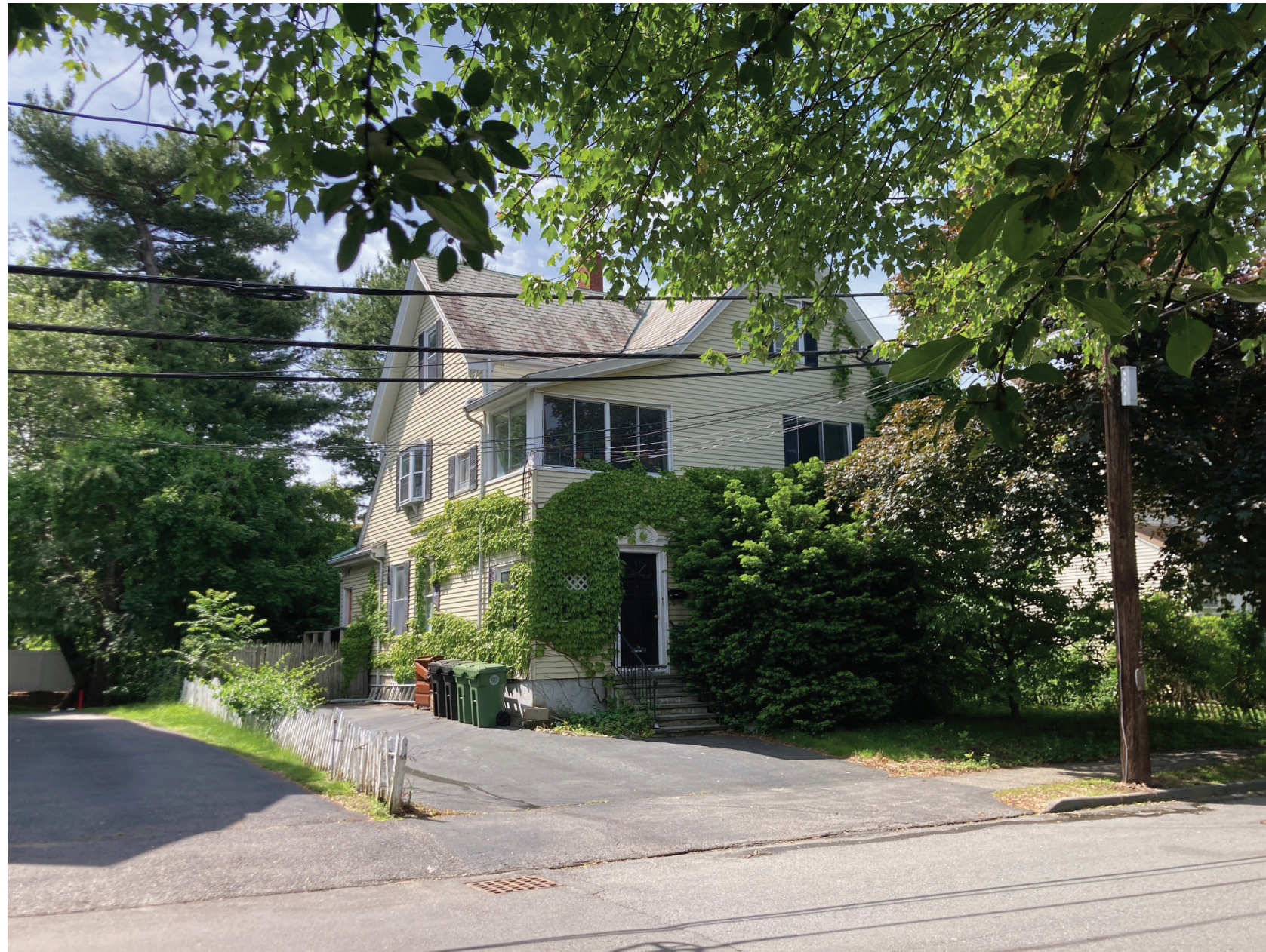
Existing building at 18 - 20 Washburn Street
