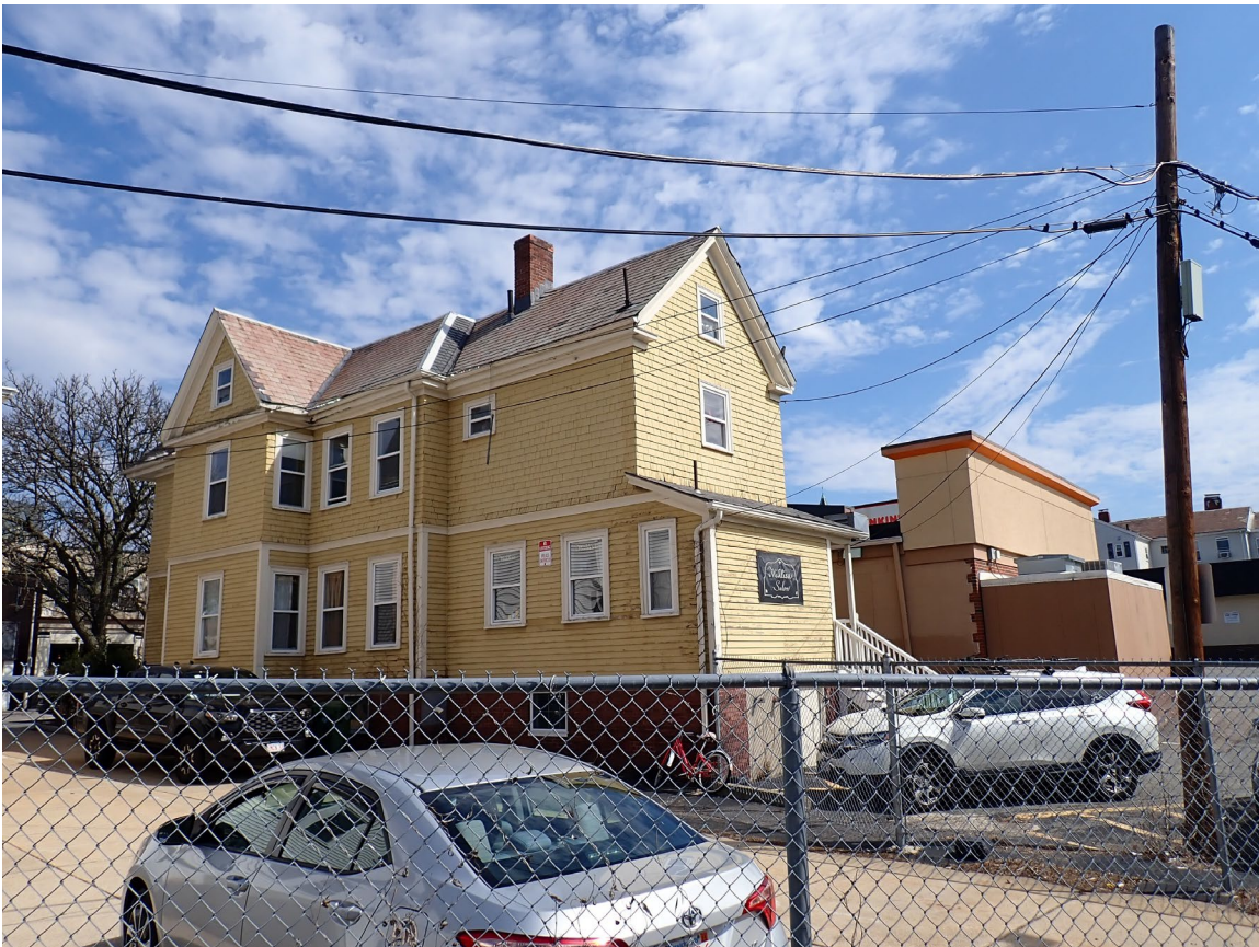
6. View of rear elevation and west elevation. 49 Mt. Auburn Street (right).
