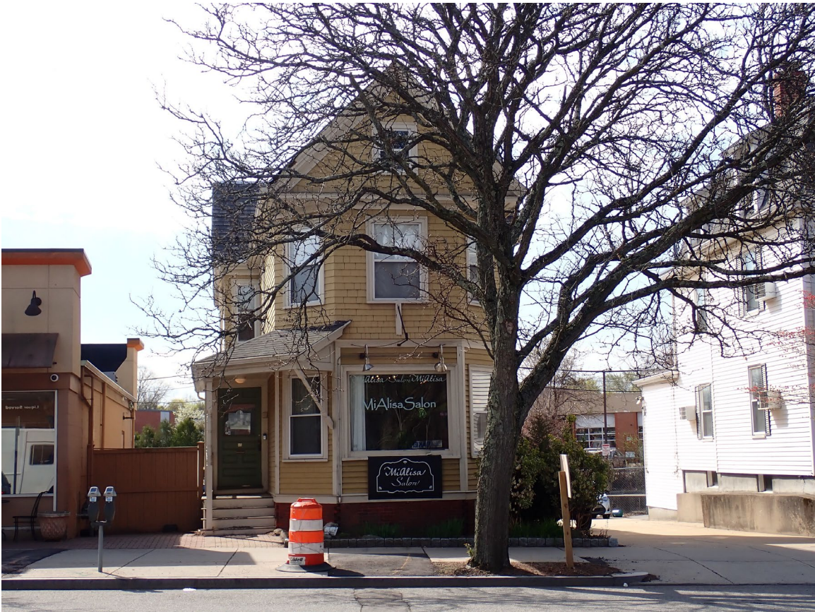
1. View of façade (north elevation) of 45 Mt. Auburn Street. Note modern display window and replacement windows. 41-43 Mt. Auburn Street (right) and 49 Mt. Auburn Street (left).
