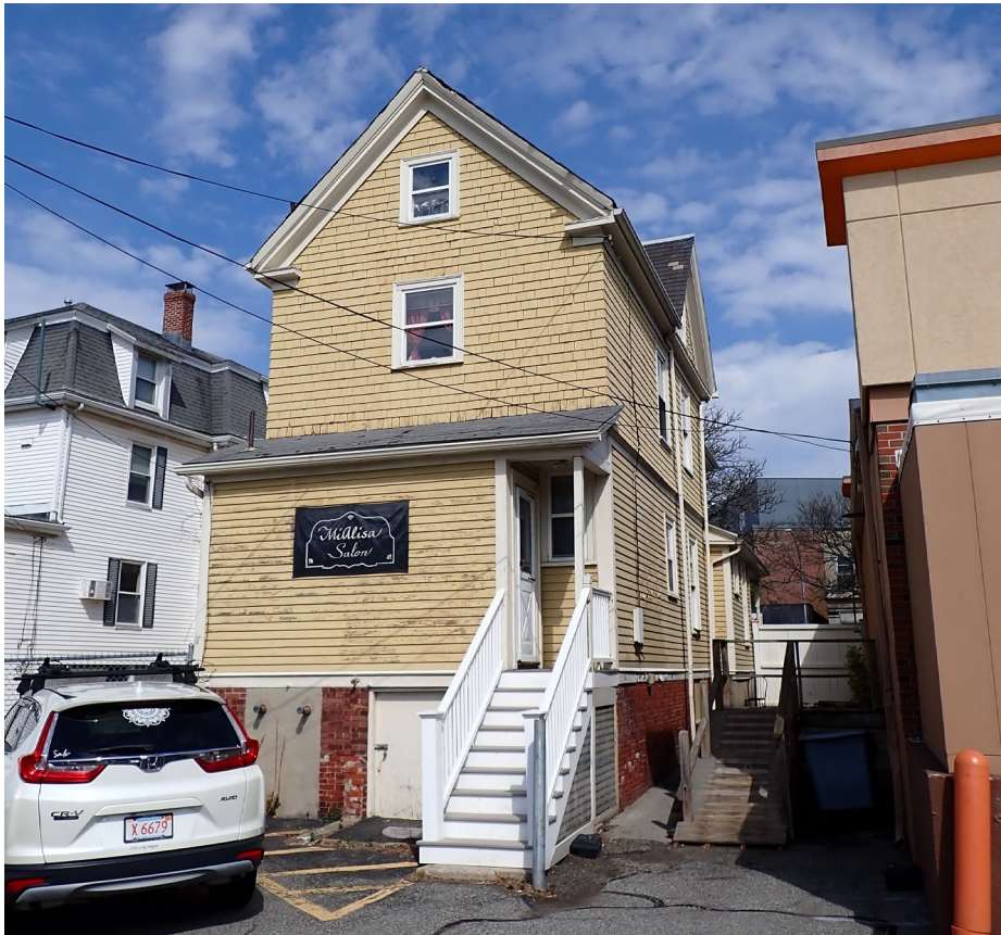
5. View of rear (south) elevation. Note infill of historic rear porch at first story. 41-43 Mt. Auburn Street (left) and 49 Mt. Auburn Street (right).
