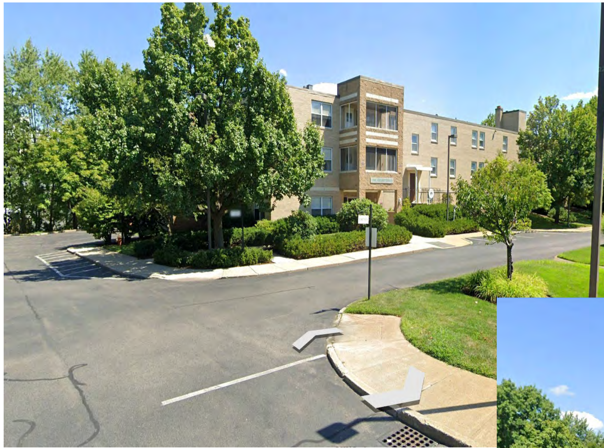
Existing view from Locust Lane looking North
