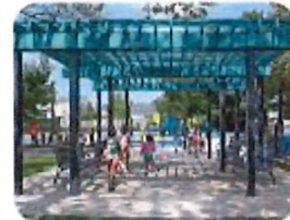
Open Roof Shade Structure
