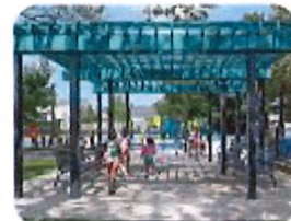
Open Roof Shade Structure
