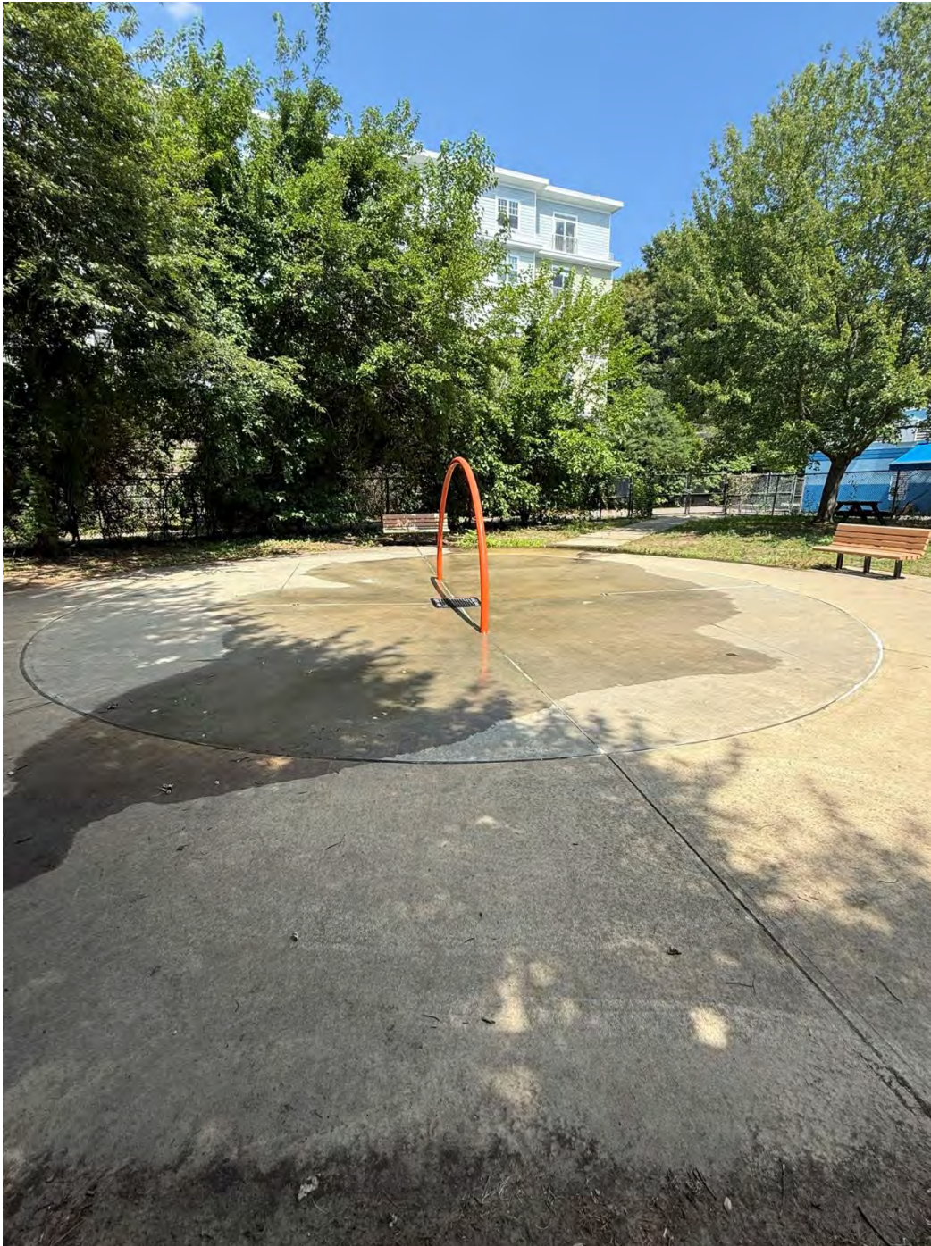
Photo 10: View of spray deck, viewing northeast.
