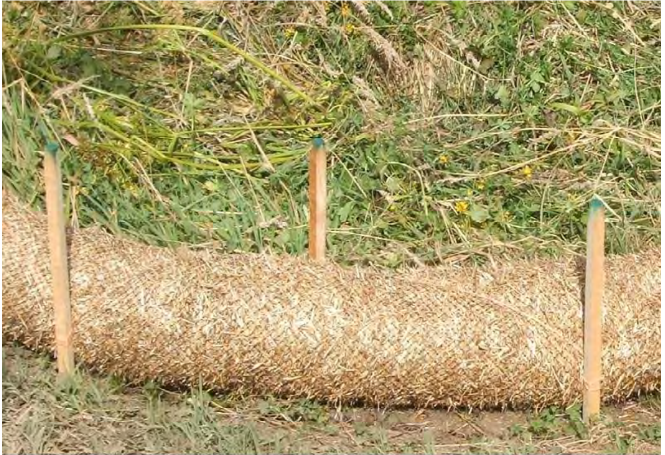
STRAW WATTLE – SHALLOW SLOPE ( \leq 4:1 ) (ALTERNATE STAKING)
