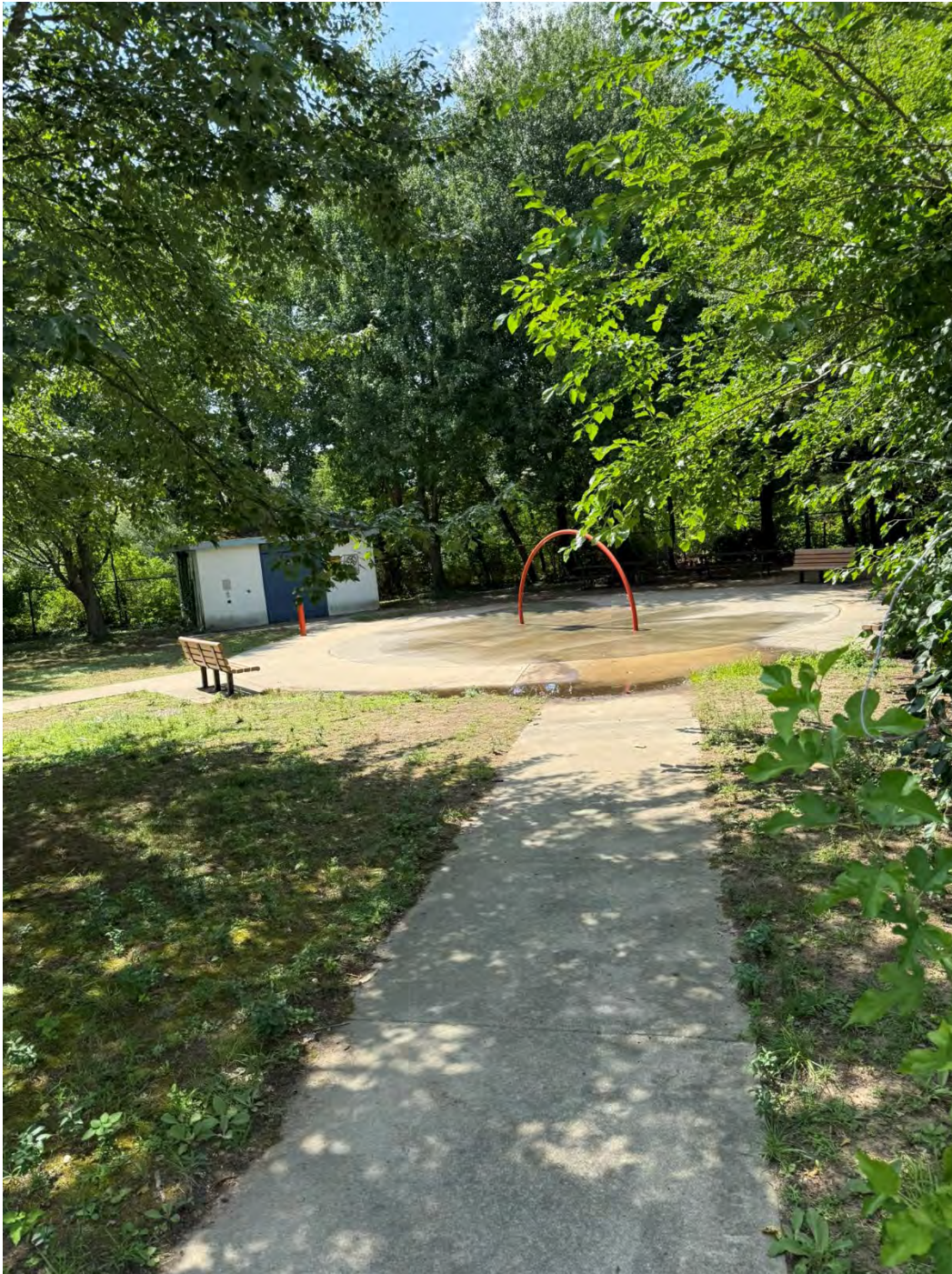
Photo 9: View of spray deck, viewing southwest.
