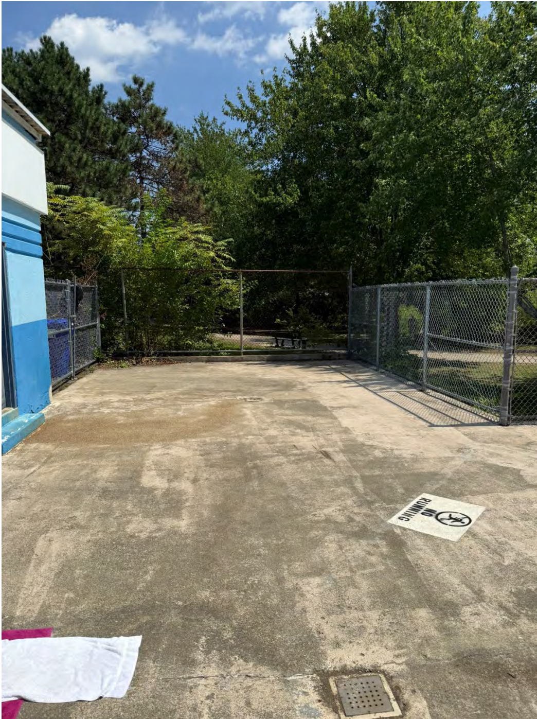
Photo 12: View of pool deck, viewing east.
