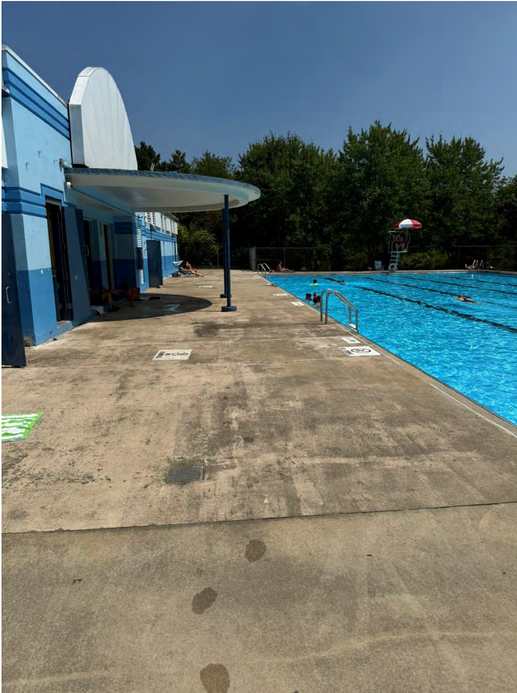
Photo 11: View of pool deck, viewing east.
