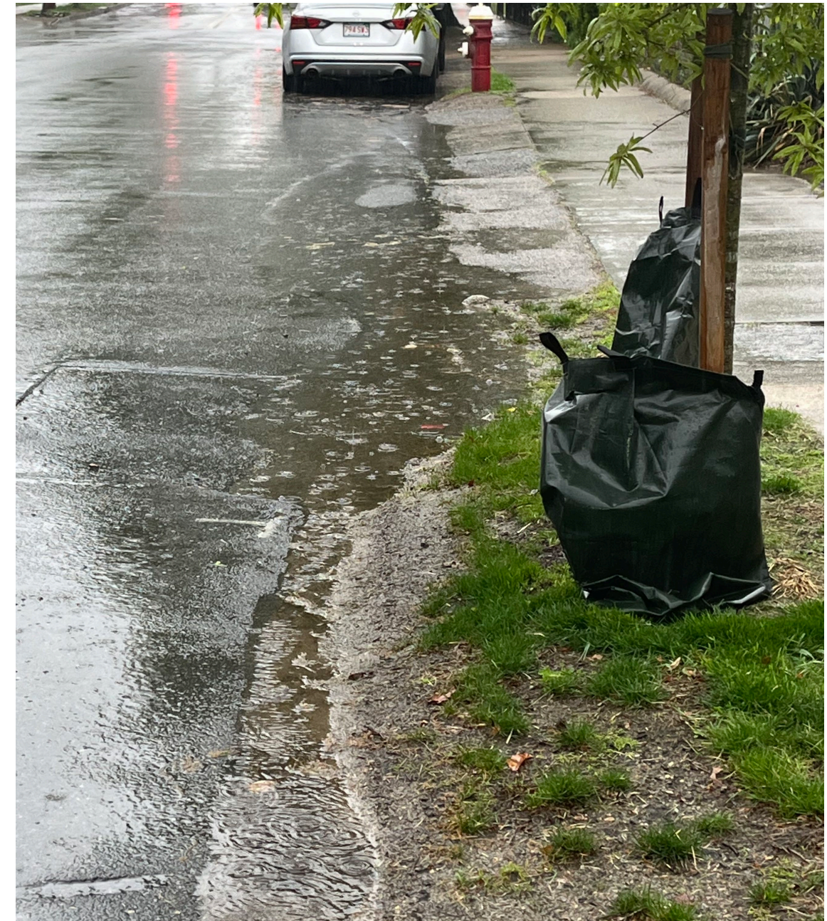
Stormwater flooding documented on Templeton Parkway, May 2025
