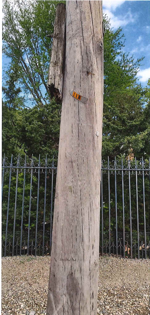
Photo 2: View of Utility Pole ID 63/18.
