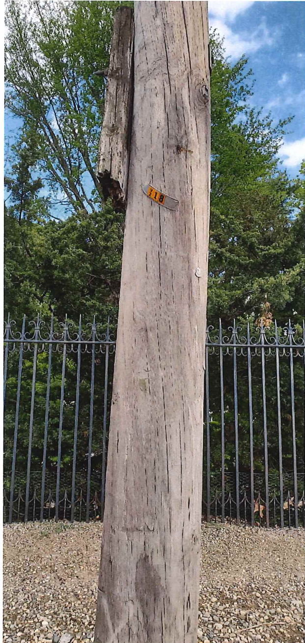
Photo 2: View of Utility Pole ID 63/18.
