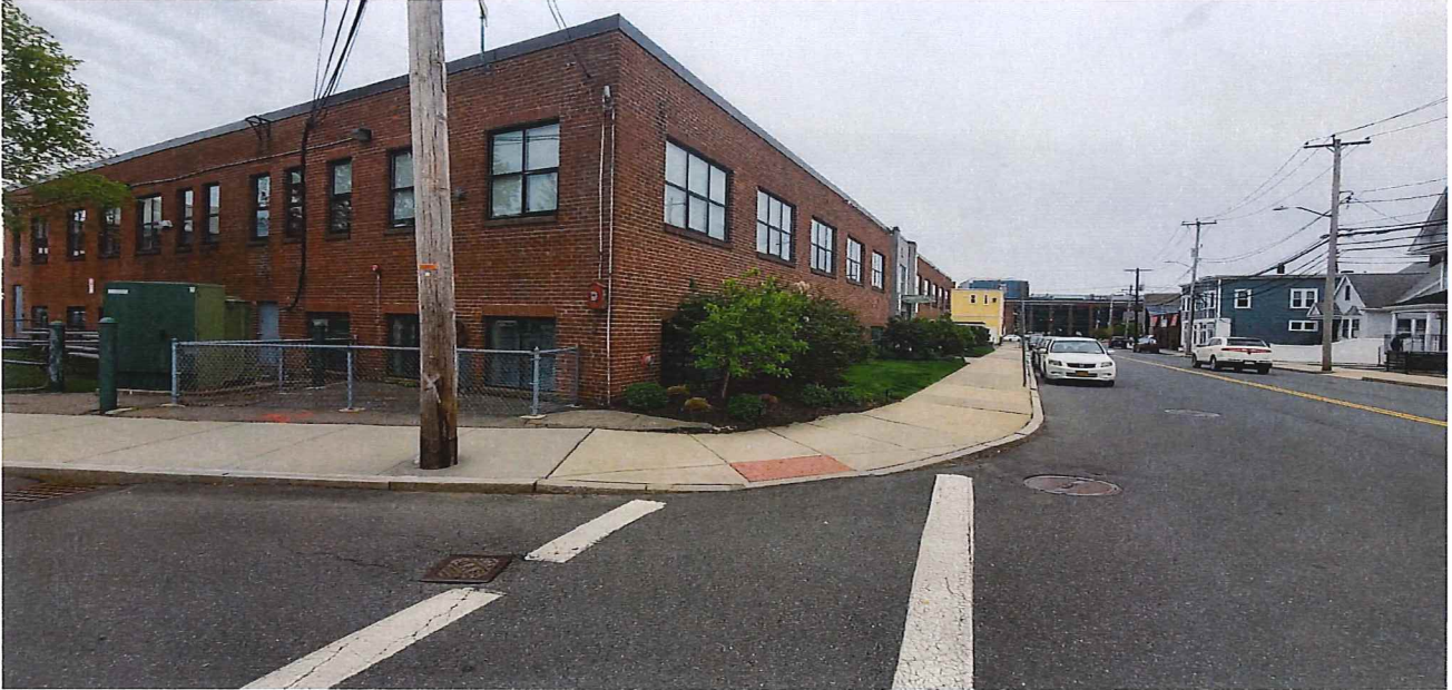
Photo 1: View of 85 School Street, manhole MH#WAT A4 and utility pole #194/11 from the corner of School Street and Cypress Street where the connection is proposed to be made from manhole MH#WAT A4 to utility pole #194/11 via two (2) new risers.
