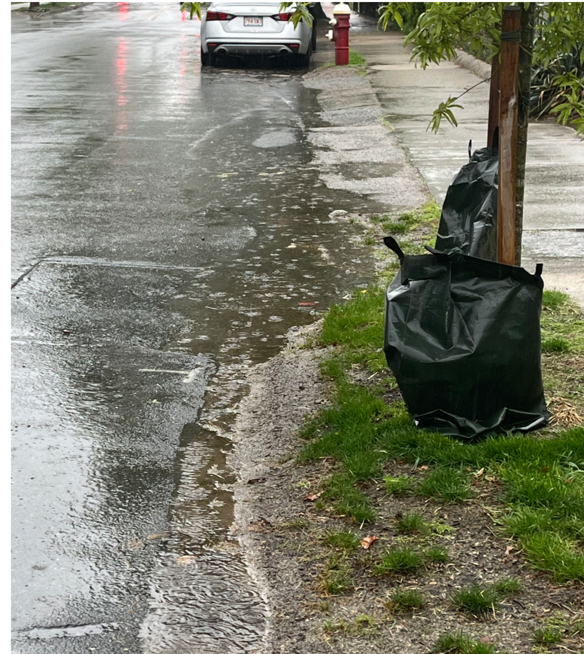
Stormwater flooding documented on Templeton Parkway, May 2025
