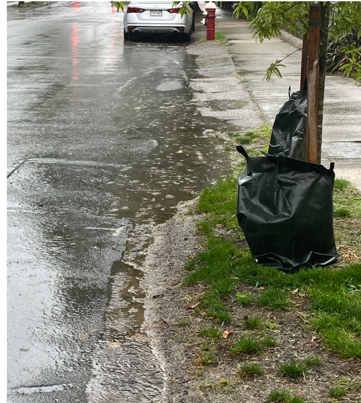
Stormwater flooding documented on Templeton Parkway, May 2025
