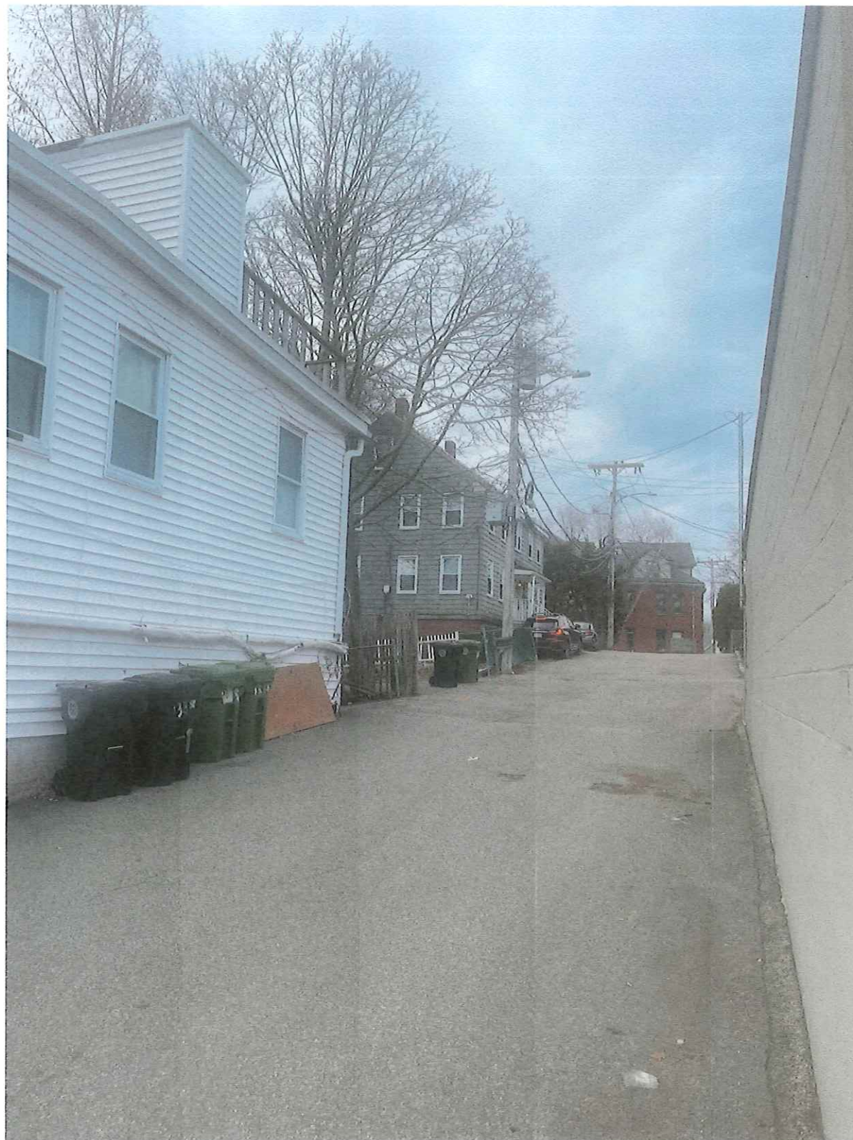
12 Church Hill Street Northerly exposure from intersection with Main Street
