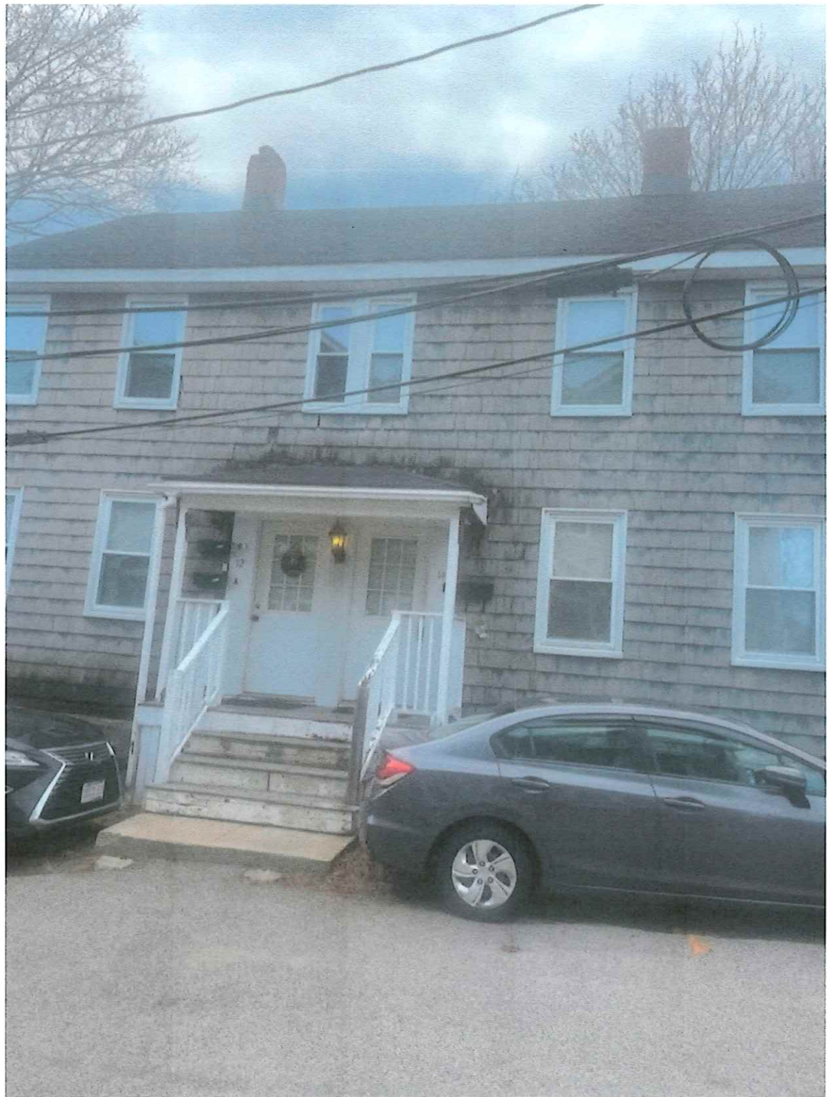
12 Church Hill Street Westerly front exposure from street
