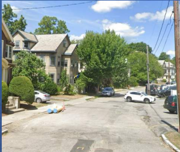
Bates Road - Before
