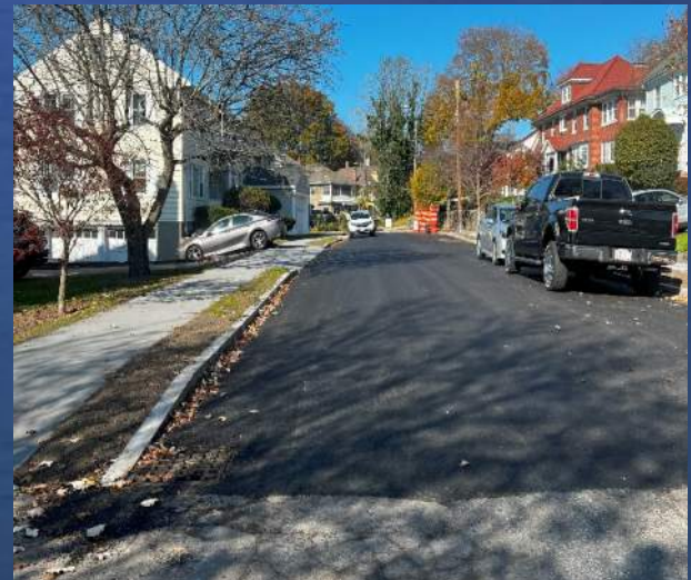
East Bates Road - After
