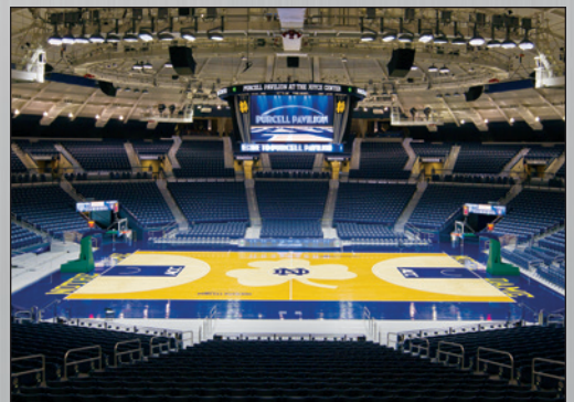
Event lighting with dimming saves energy for high-usage, multi-use venues.
