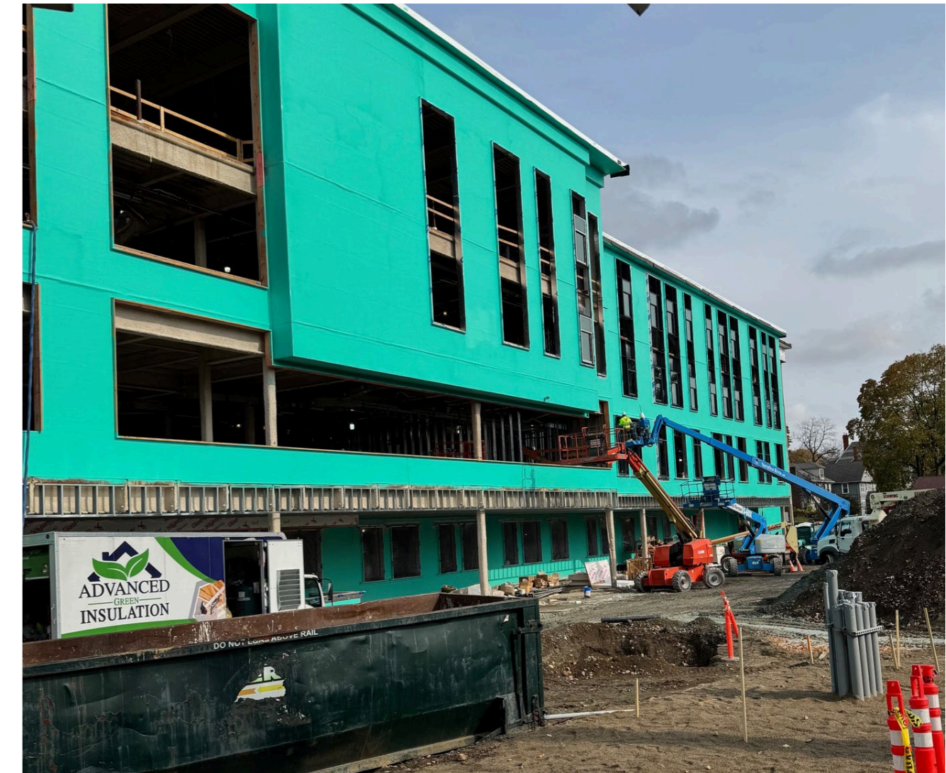
Watertown's LEED Platinum high school building under construction
