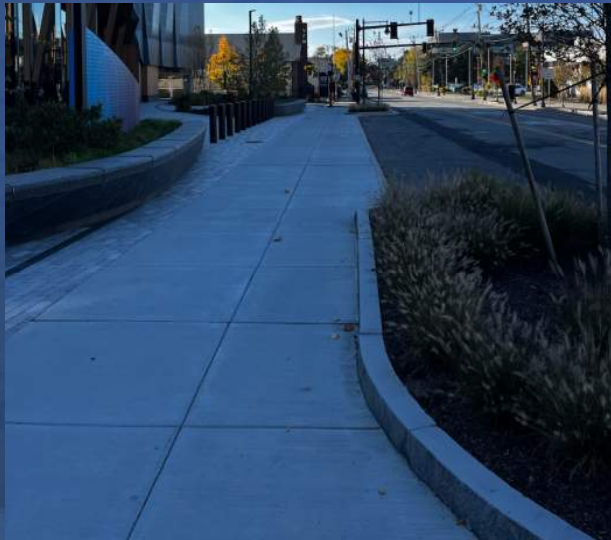
Arsenal St Phase D - After
