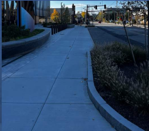
Arsenal St Phase D - After
