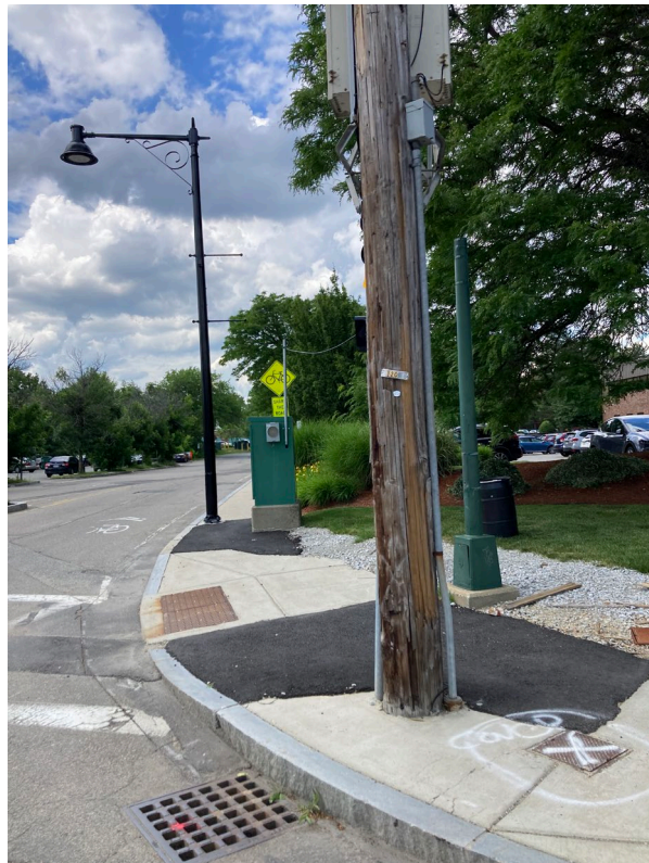
View of UP#5/20 on Arsenal Street facing northwest where conduit is proposed to be installed.
