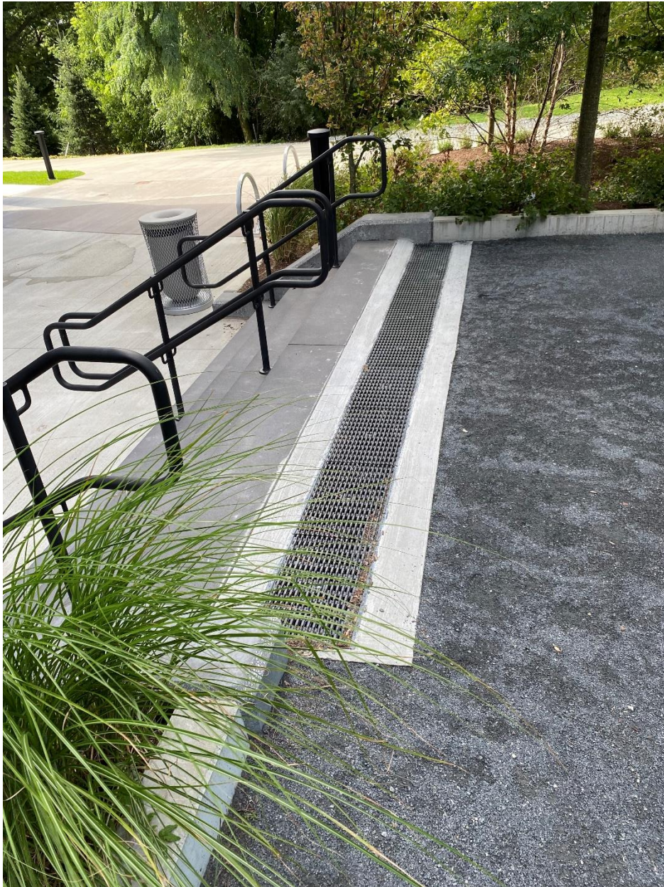
Photo 1: Additional trench drain at the top of the stairs.
