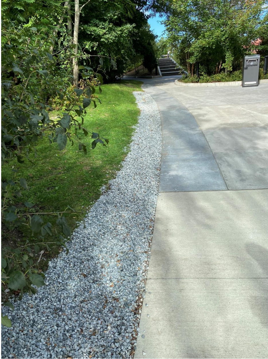
Photo 3: Crushed stone infiltration trench along the south pathway to prevent erosion.
