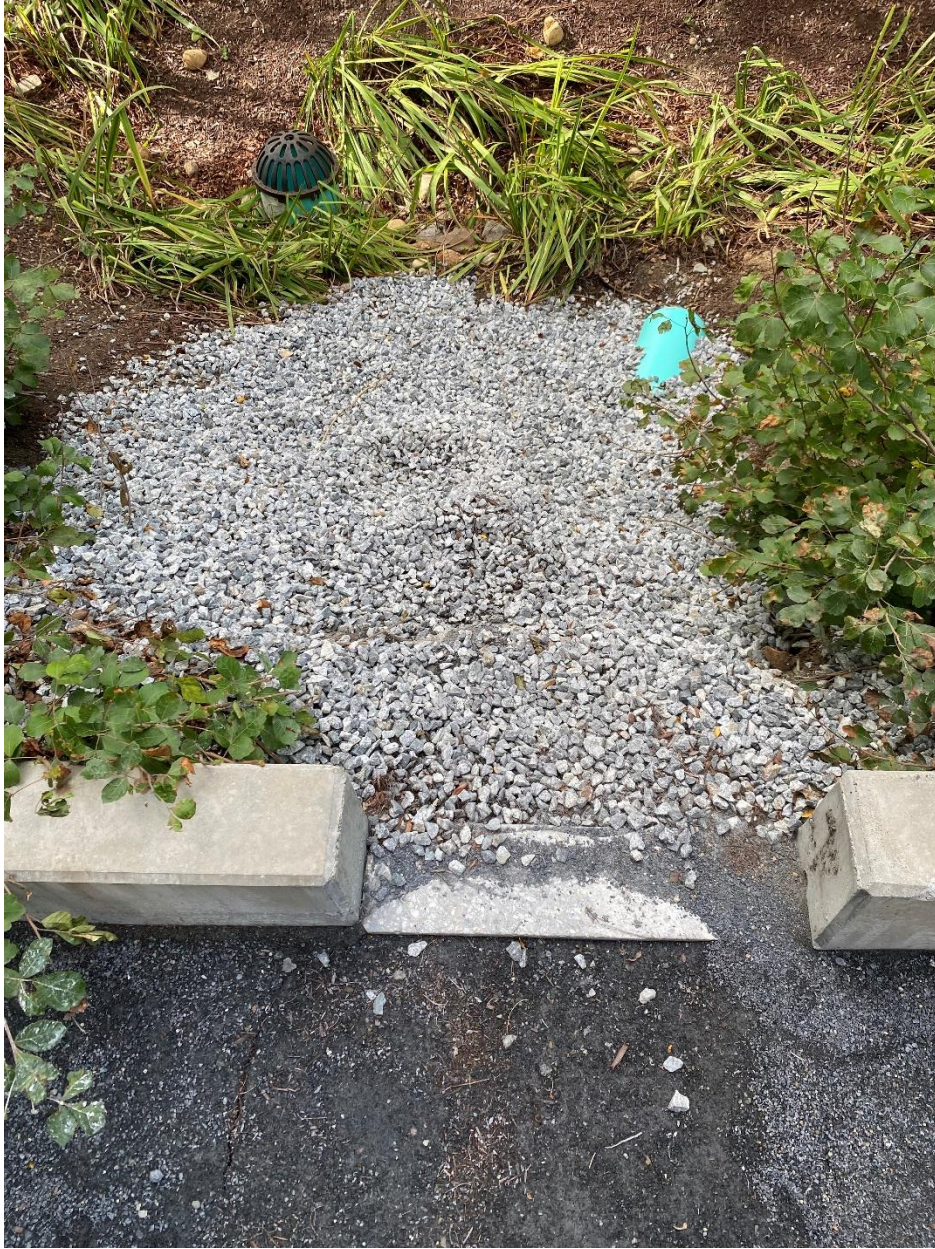
Photo 4: Crushed stone placed at the outlet for the rain garden (to be replaced with rounded stone once delivered).
