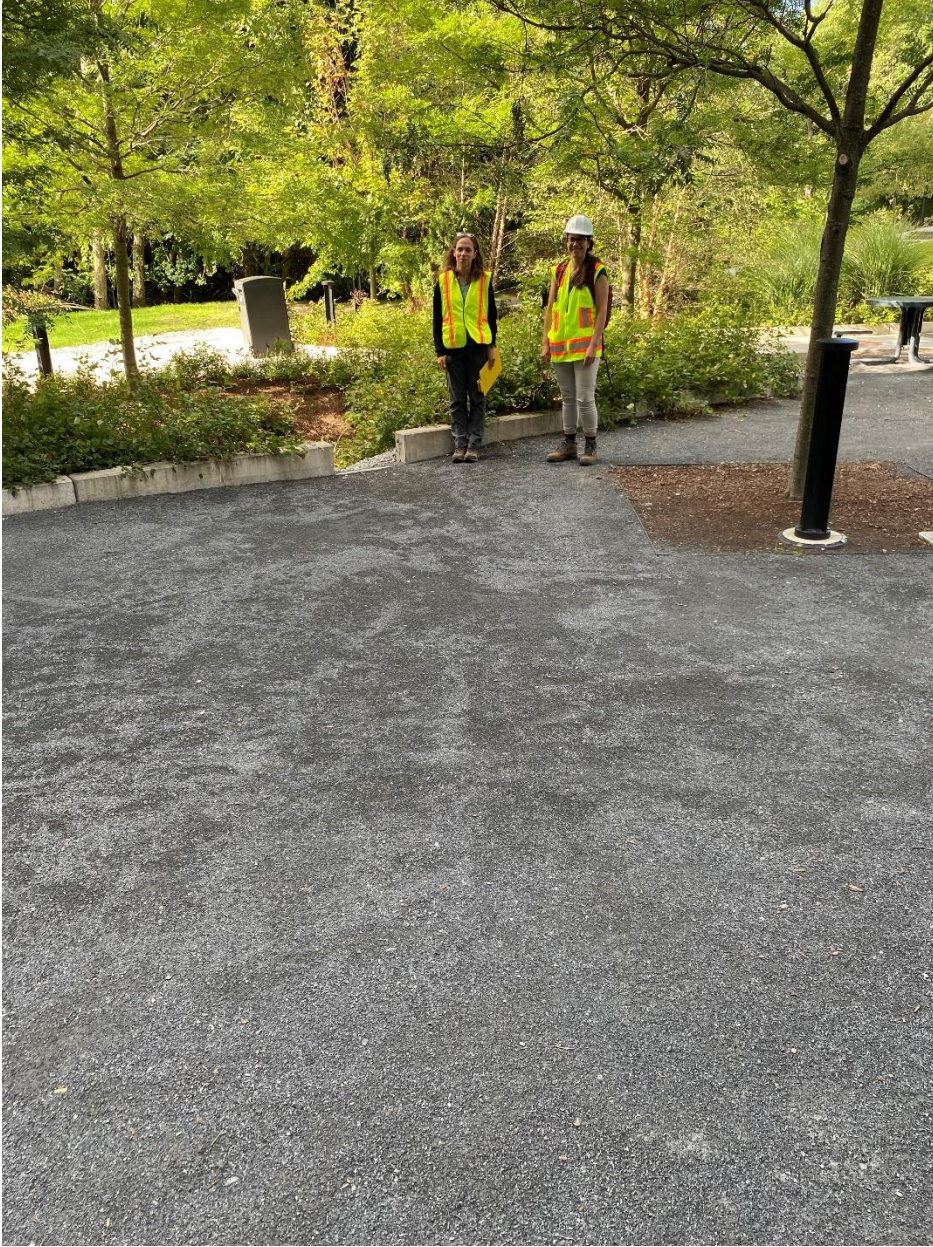
Photo 2: Regrading of the stone dust within an area of the Bosque.
