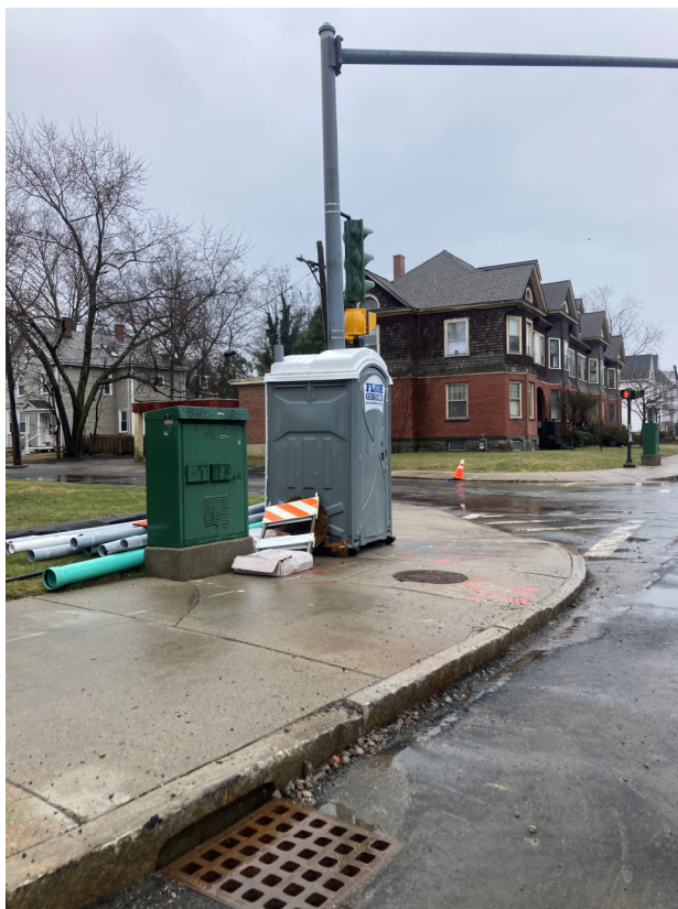
View of the intersection of Irving Street and Mount Auburn Street from the approximate location of the MWRA meter pedestal facing southwest.
