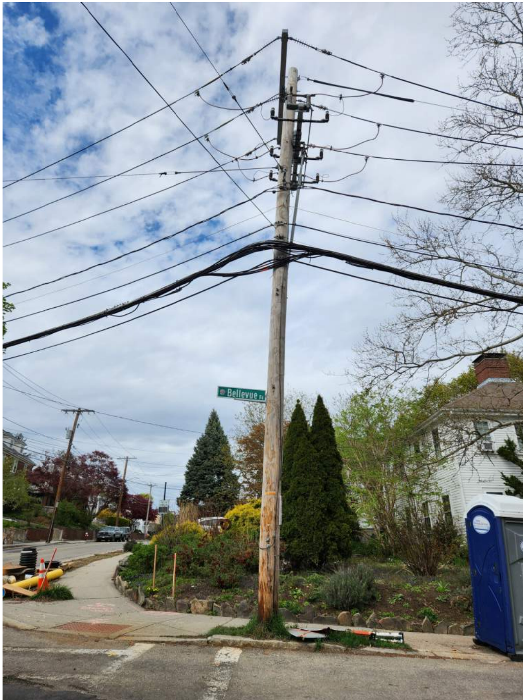
View of utility pole #12/11 on the corner of Bellevue Road and Common Street facing north.
