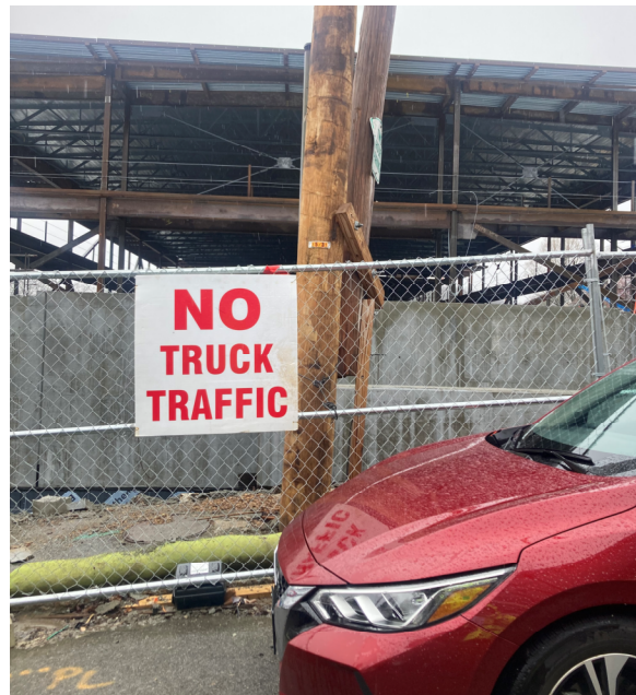
View of UP#31/5 facing 50 Columbia Street where conduit is proposed to be installed.
