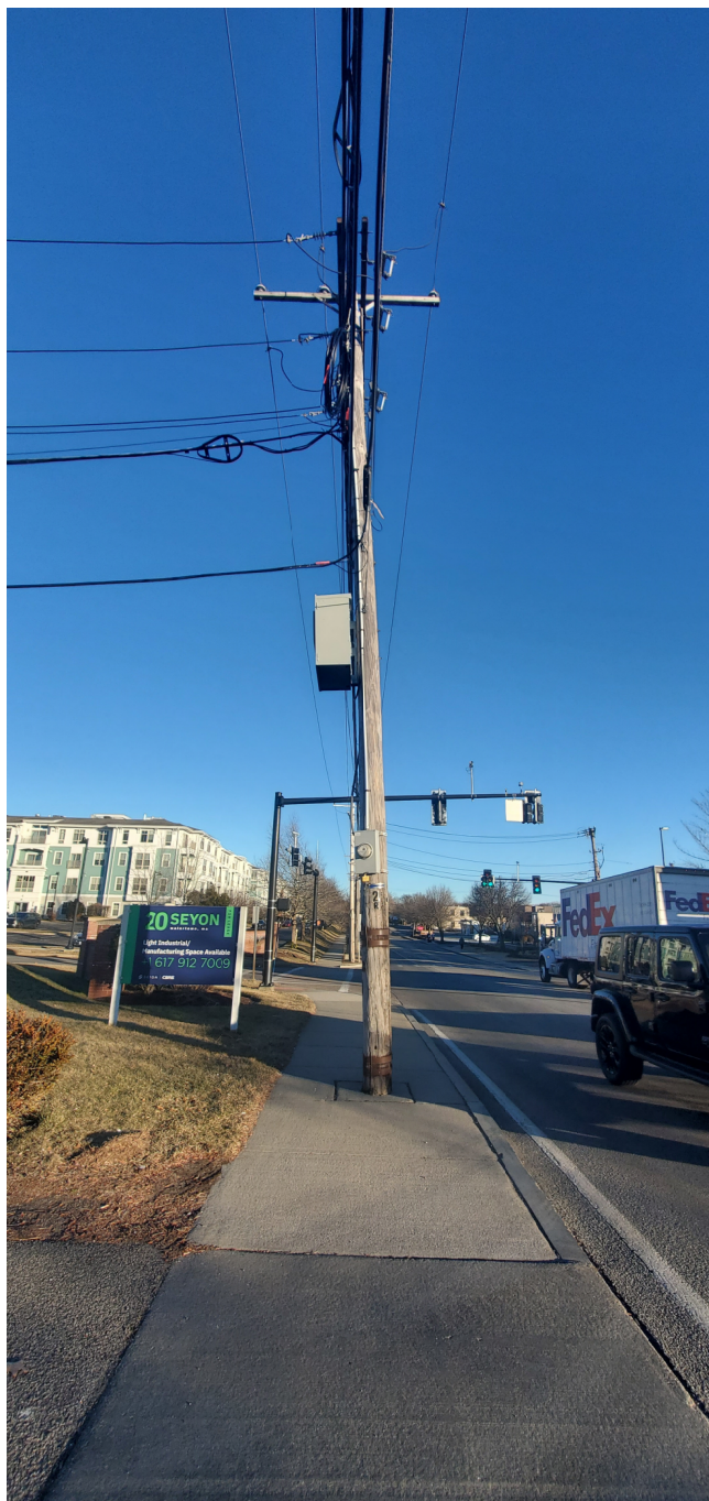
View of Utility Pole #16/78 and associated sidewalk facing east.
