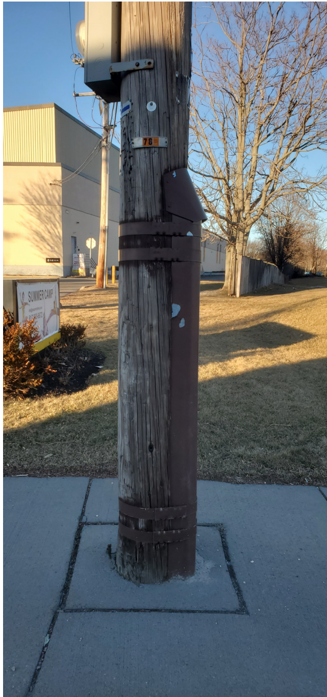
View of Utility Pole #16/78 from Pleasant Street facing the property at 10-30 Manley Way.
