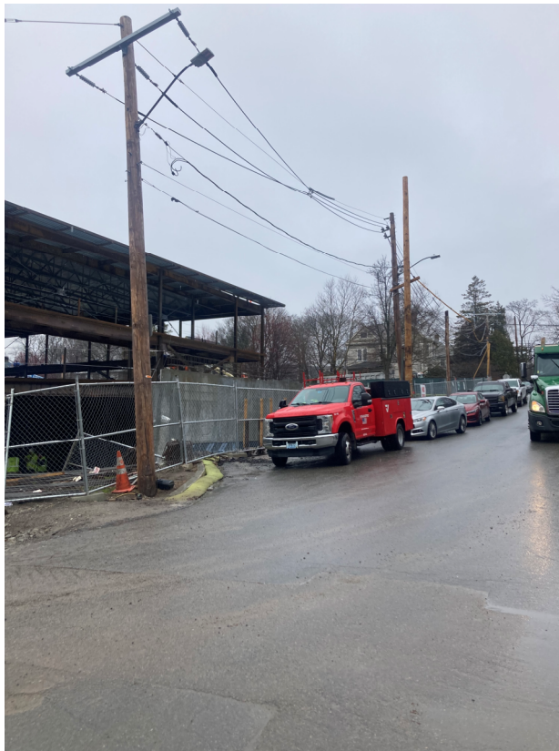
View of Barnard Avenue from UP#31/4 facing north.
