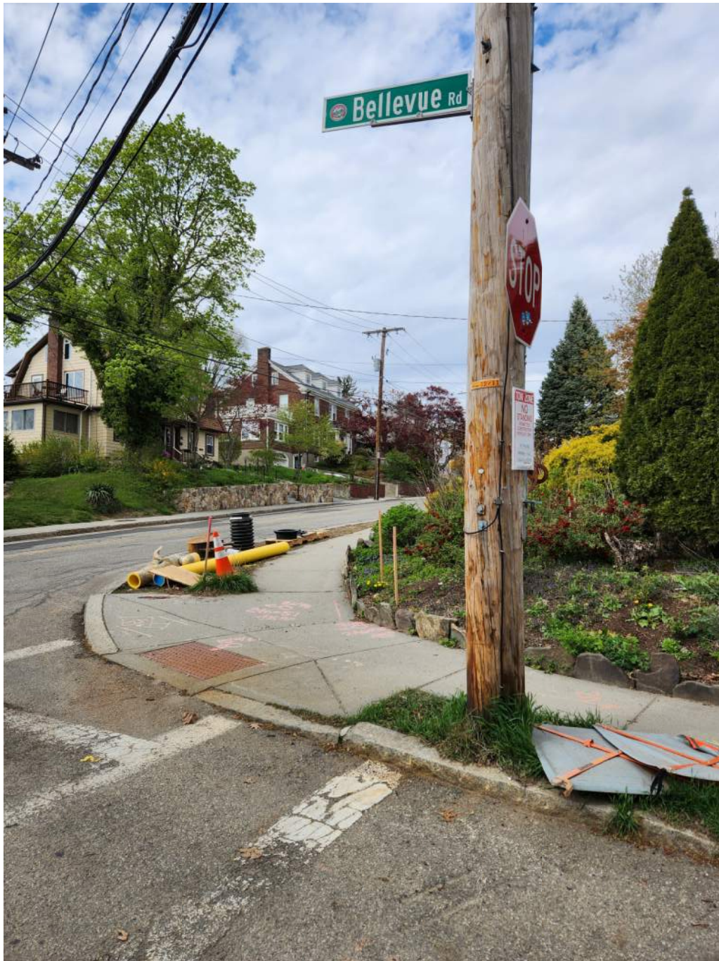
View of utility pole #12/11 and work areap on the corner of Bellevue Road and Common Street facing north.
