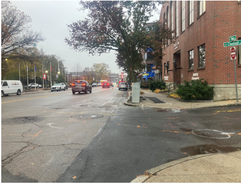
View of Main Street from the intersection of Main Street and Chestnut Street facing northeast.
