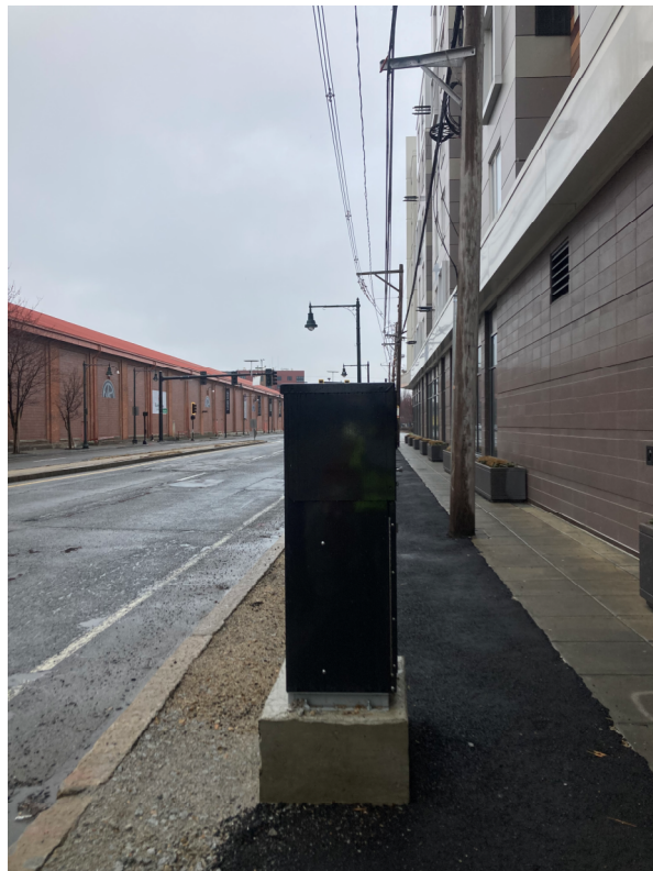
View of Arsenal Street from proposed street light control cabinet facing west.
