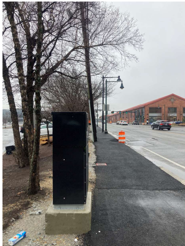
View of Arsenal Street from the proposed street light control cabinet facing east.
