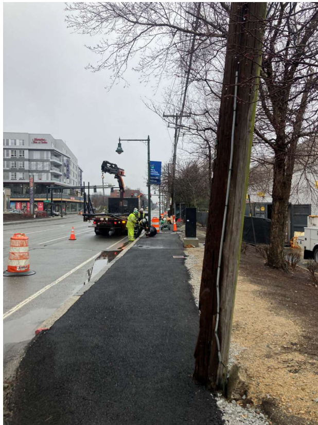
View of Arsenal Street from utility pole #13 facing west.
