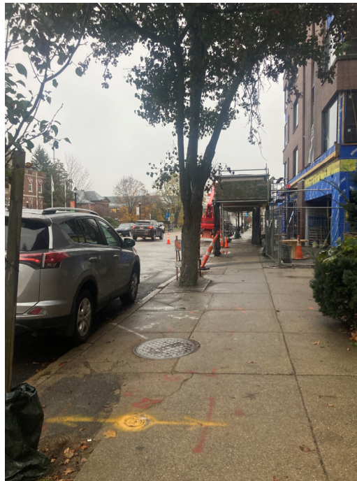
View of Main Street from MH14667 facing southeast.
