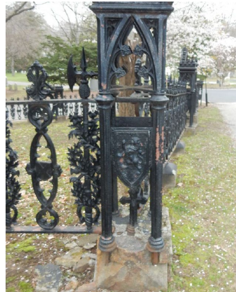
Scots Charitable Society Plot Fence Deterioration of Base
