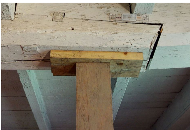
Support and crack monitor
