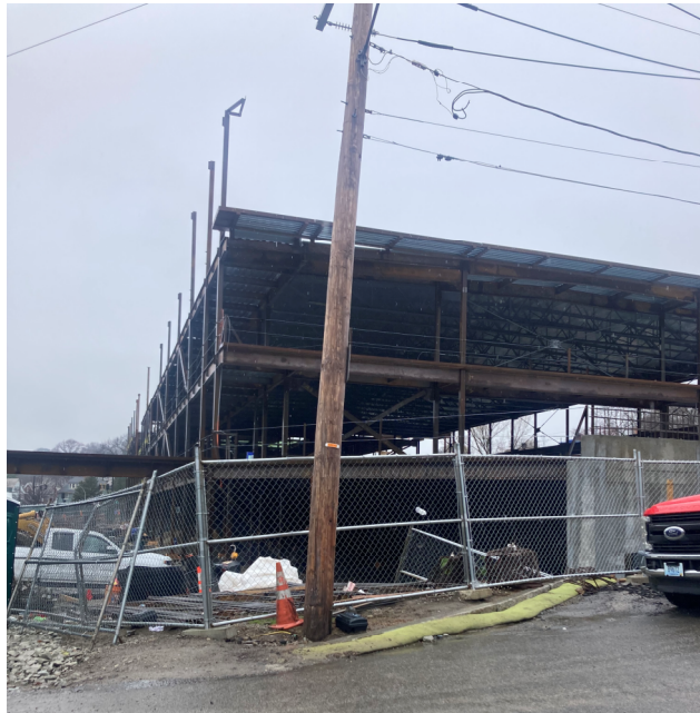
View of UP#31/4 facing 50 Columbia Street where conduit is proposed to be installed.
