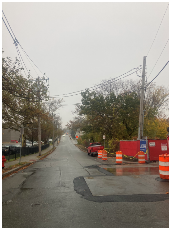
View of Elm Street facing westward away from Arsenal Street where new conduit is proposed.
