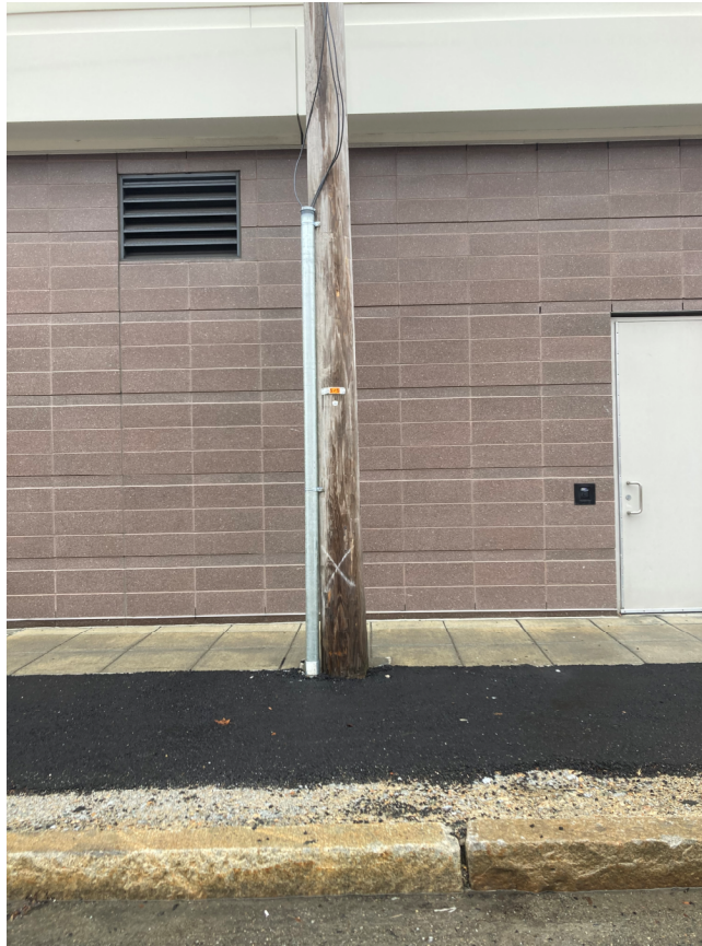
View of utility pole #5/5 where conduit is proposed to be installed facing 570 Arsenal Street.
