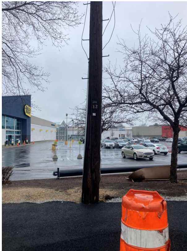
View of utility pole #13 facing 550 Arsenal Street where conduit is proposed to be installed.
