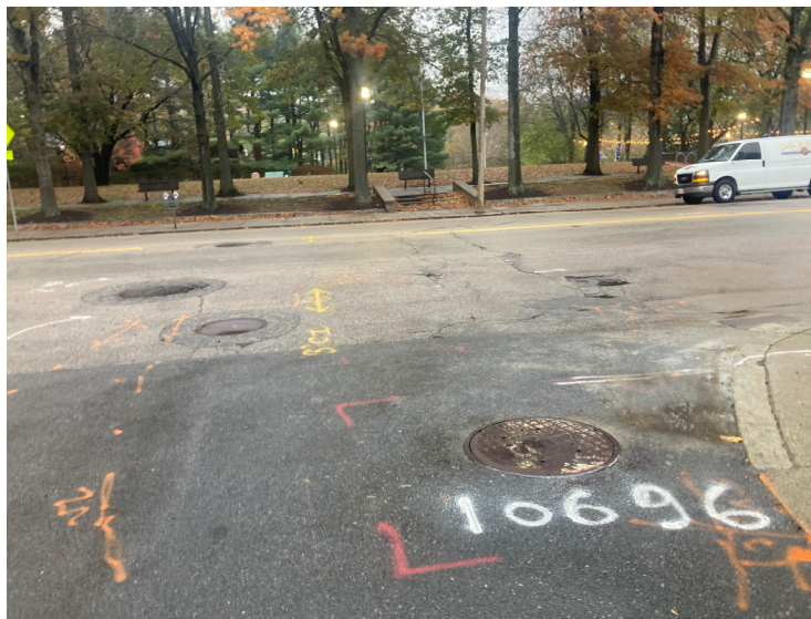
View of the intersection of Main Street and Chestnut Street from MH10696 facing northeast where service will be pulled from.
